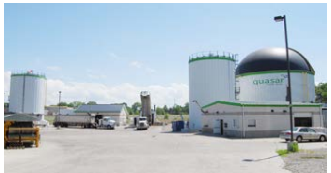
Collinwood BioEnergy - Cleveland, OH Owned by quasar energy group
