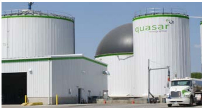
Central Ohio BioEnergy - Columbus, OH In Collaboration with SWACO & Kurtz Bros., Inc.
