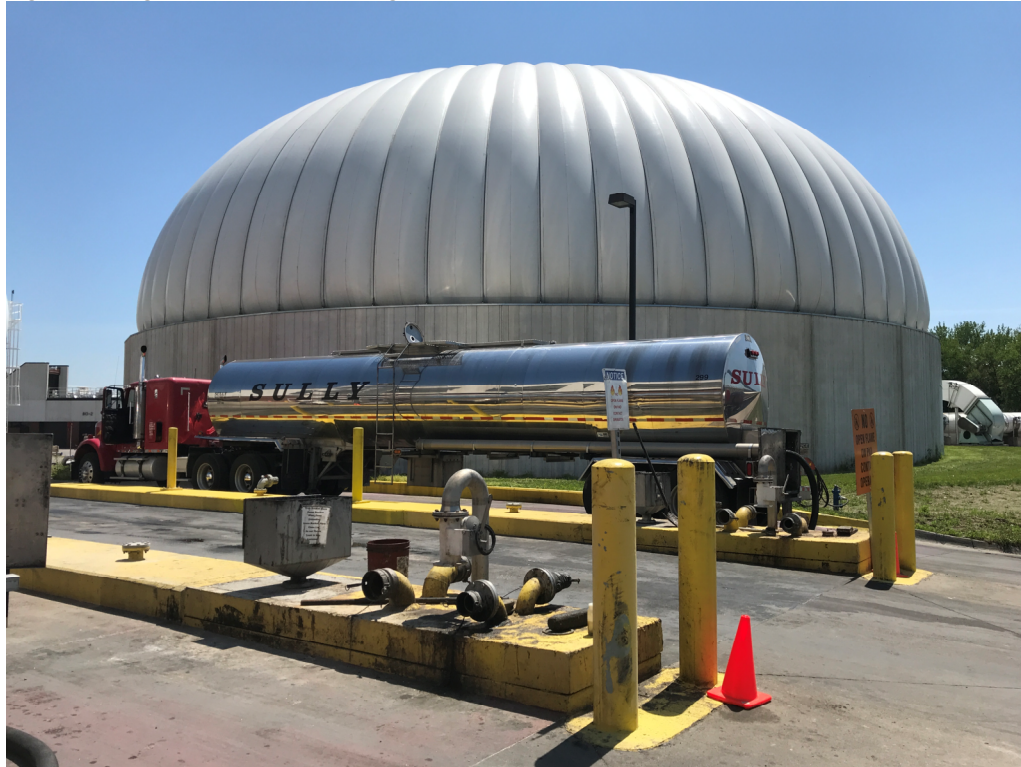
Figure 5: Organic Waste Receiving Station at Des Moines WRF
