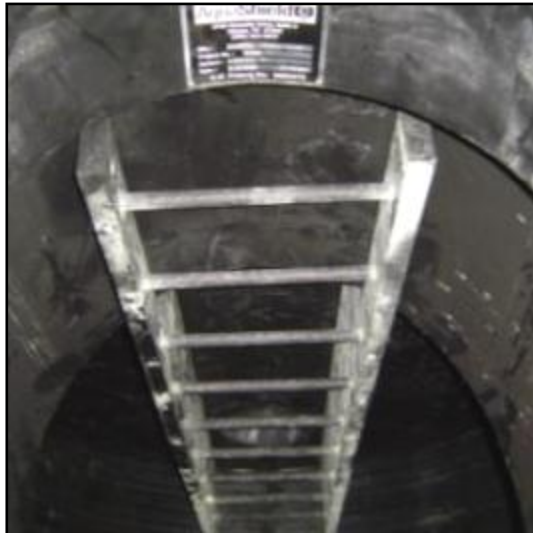
A permanent ingress/egress ladder provides access to filtration chamber. Note metal product identification plate above ladder.
