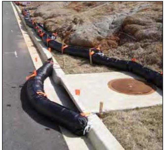
Sediment Tube used as Inlet Protection
