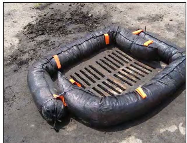
Sediment Tube used as Inlet Protection
