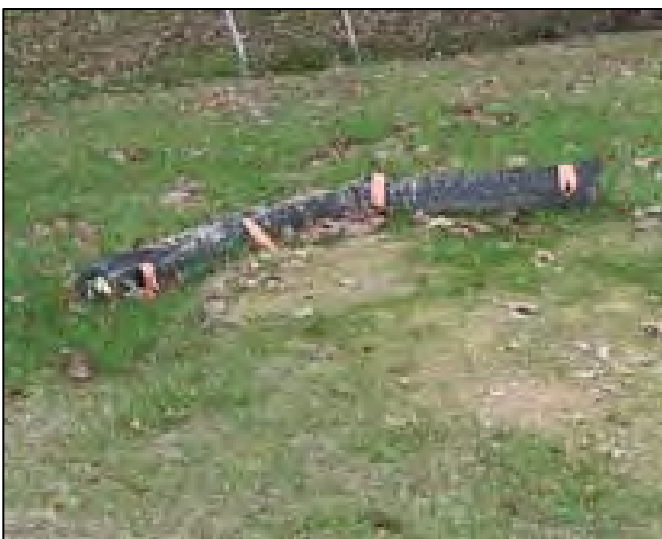
Sediment Tube used on Open Ground
