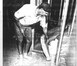
Homearama builder John Harris pulls back insulation to reveal spray-in foam Insultighter more efficient home by preventing heat and cooling losses through cracks.
