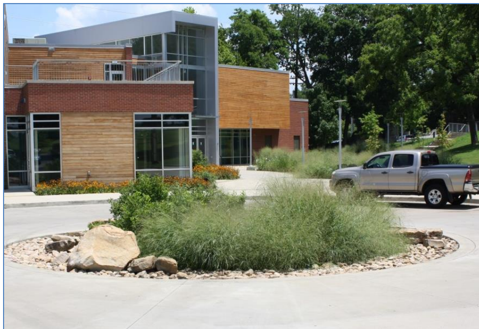
Figure 37. Installation of bioretention at McCabe Community Center.
