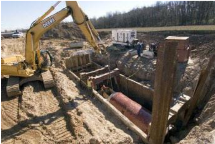
Figure 33. This picture shows a new conveyance being installed that will increase carrying capacity of undersized sewer mains.
