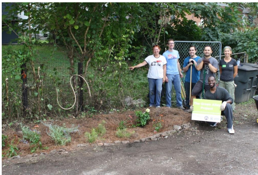
Figure 42. Volunteers working on installation of a Green Alley rain garden
