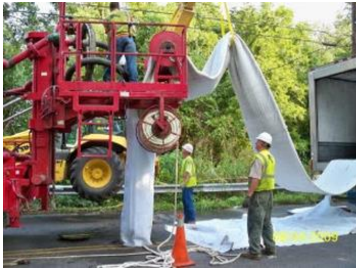
Figure 32. This picture shows a sewer lining project that is used to reduce infiltration into the sewers.
