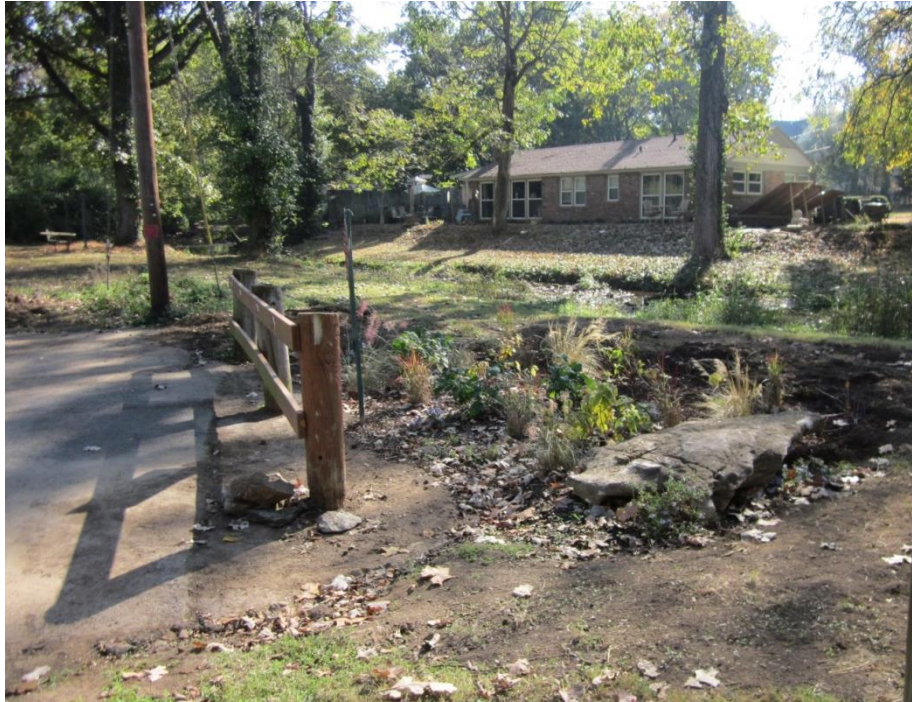
Figure 43. Recent installation of a rain garden at the end of Hilldale Drive.
