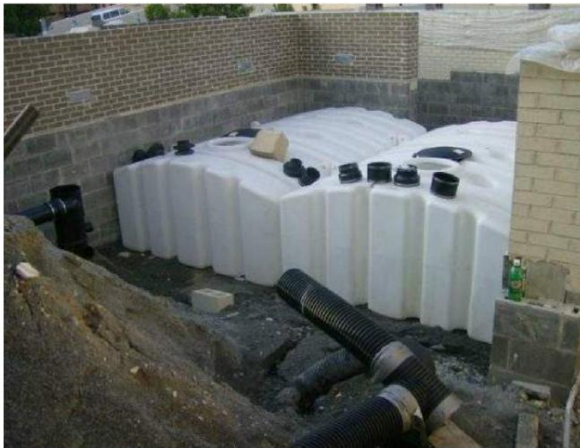
Figure 10.5. Example of two Polyethylene Cisterns (Source: VADCR, 2011)
