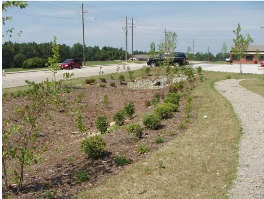
Filter strip surrounding bioretention cell, Fort Bragg, NC. (Source: N.Weinstein, LIDC)
