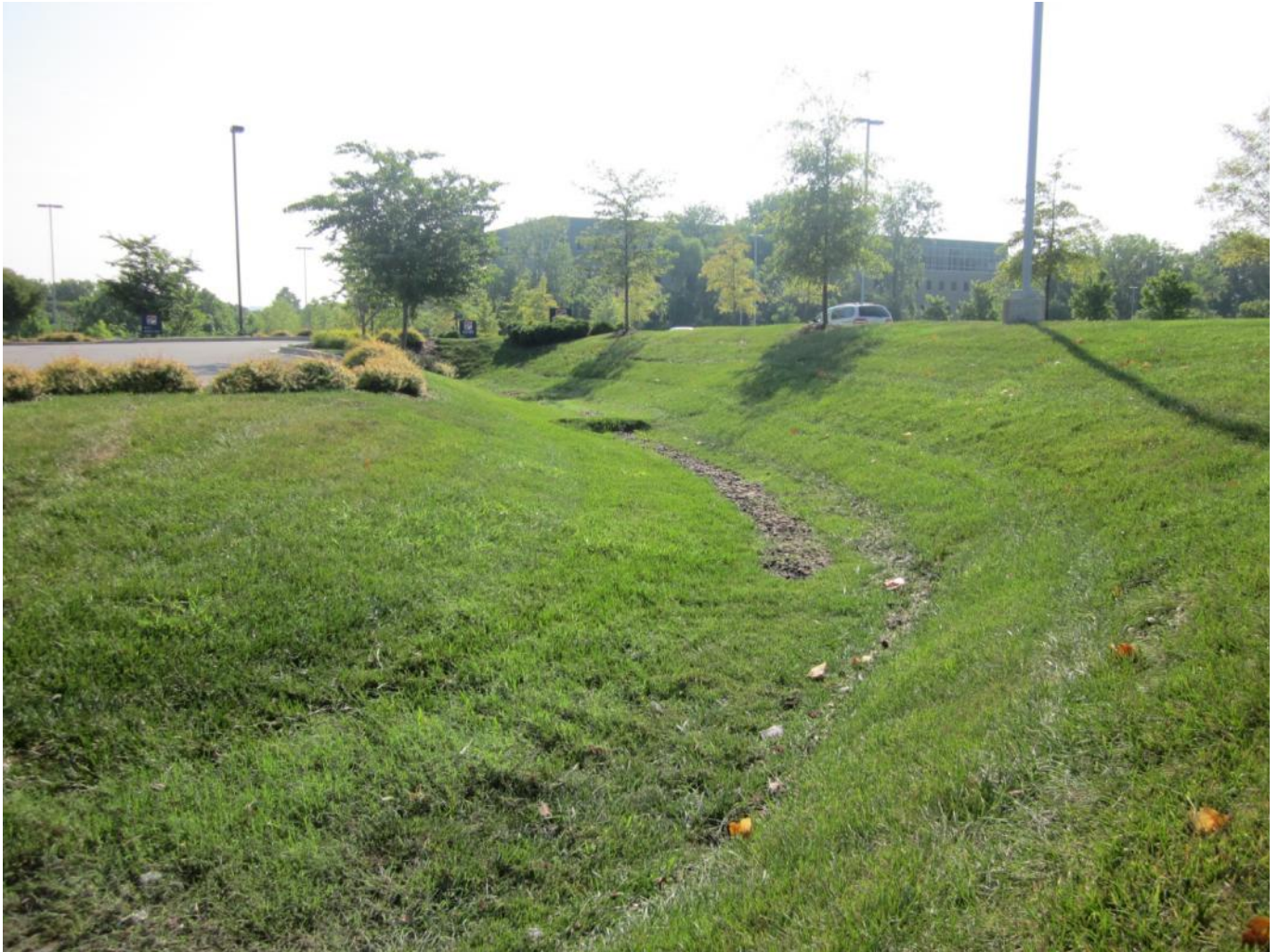
Figure 7.1: Typical Grass Channel Rosa Parks Boulevard, Nashville, TN
