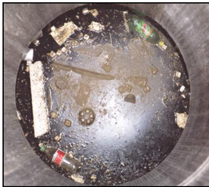
Floatable trash & debris in the Aqua-Swirl ®
