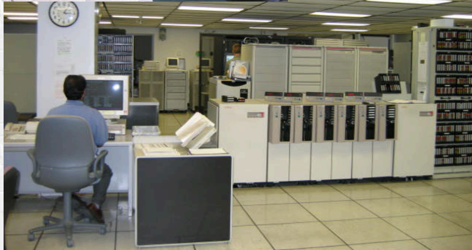
MNPD Data Center
