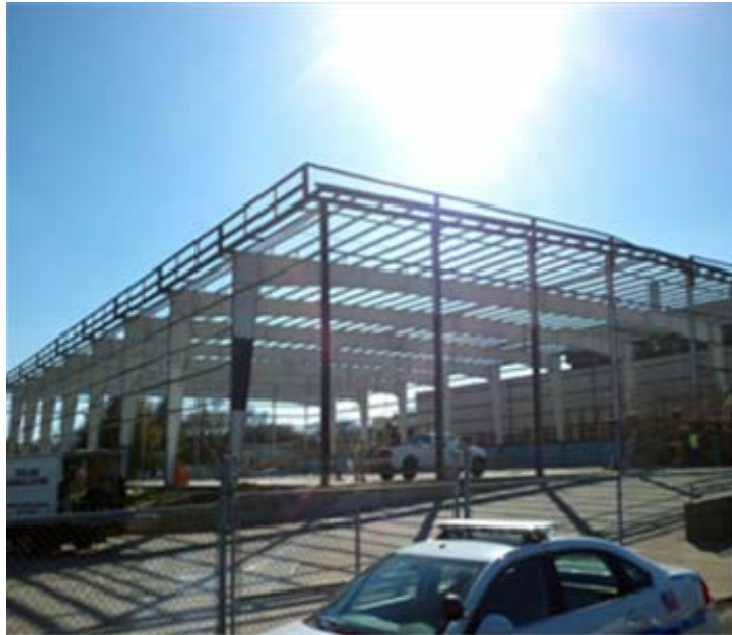
Madison Precinct and crime lab under construction.
