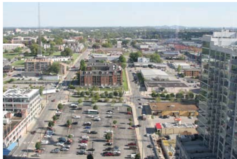
SURFACE PARKING BETWEEN SECOND AND THIRD AVENUES AT KVB
