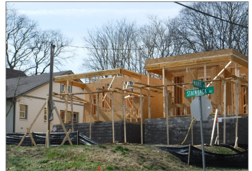
New construction in progress on Stainback Avenue
