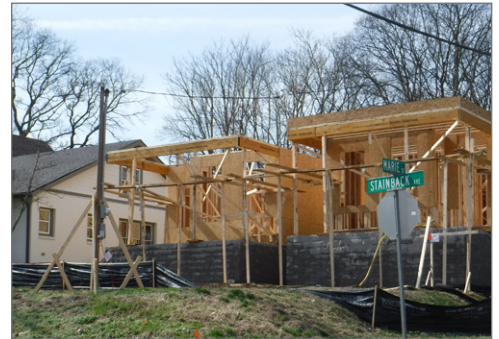
New construction in progress on Stainback Avenue
