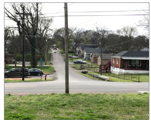
Gatewood Avenue is one of many study area streets without sidewalks
