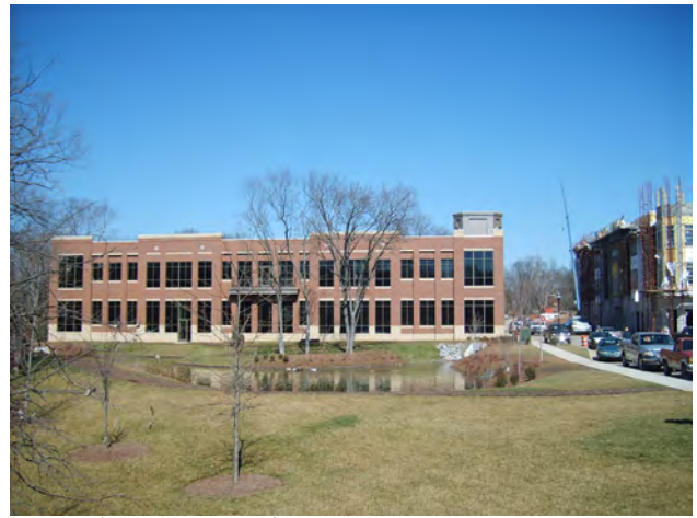
Regional Detention Pond
