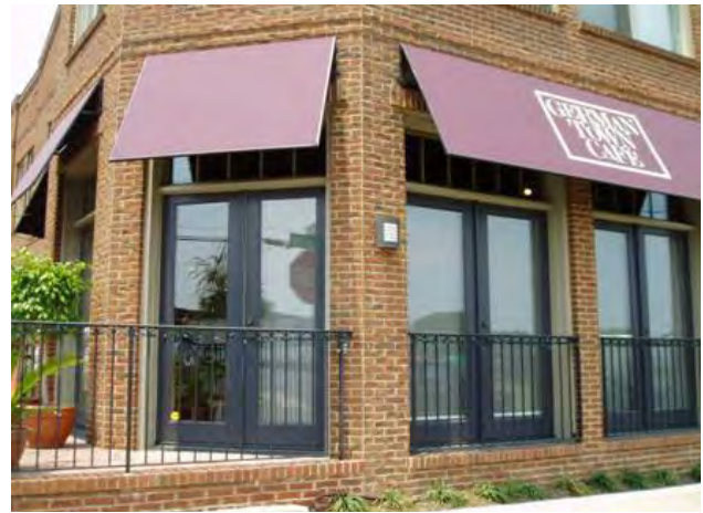
Signage incorporated into an awning.
