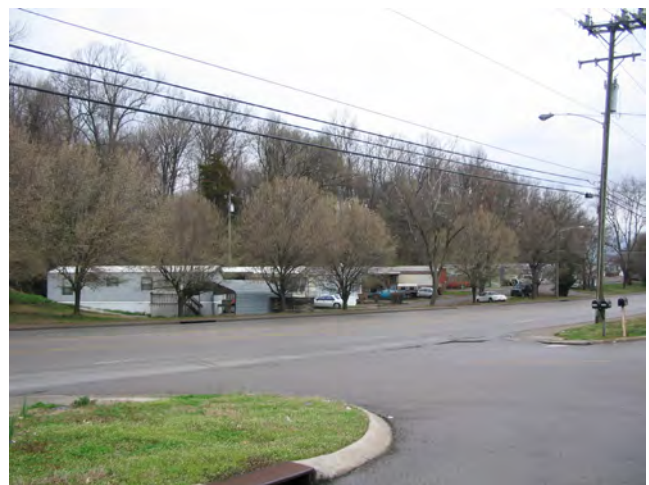
Existing mobile homes located within the flood plain along Antioch Pike.
