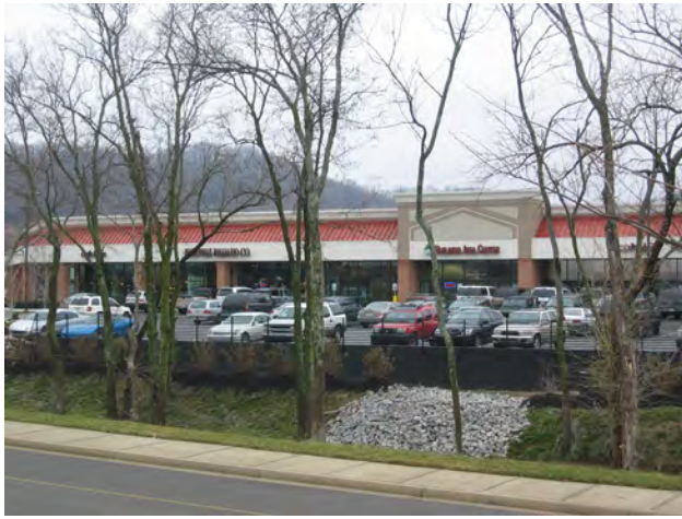
Vegetative buffer that preserves existing trees and screens parking areas that face a public street.
