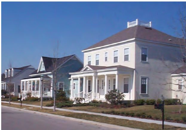
Single-family residential sited with consistent setbacks to maintain a consistent building form and rhythm along the street.
