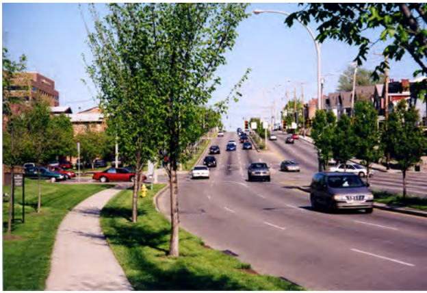
Arterial road similar to Antioch Pike with a median and streetscape design that is pedestrian-friendly with tree plantings located along the road.
