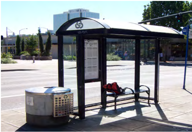
Public transit stop that provides shelter and seating.
