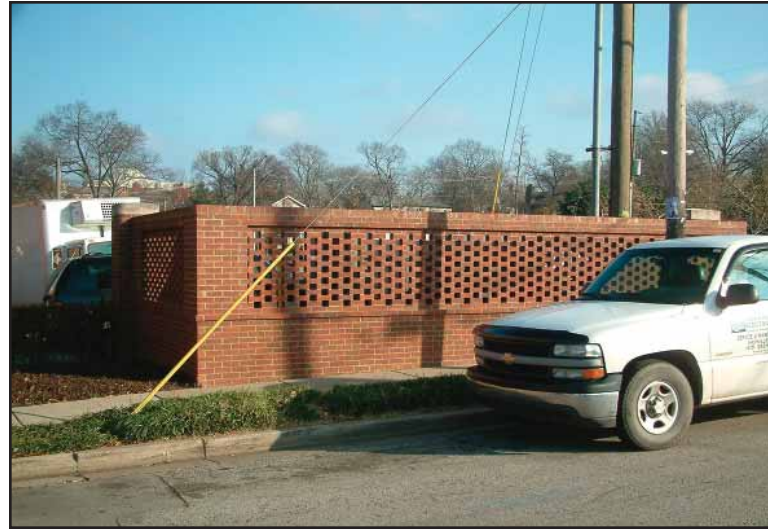
Photo 10.1—Masonry screen wall at ground level mechanical equipment.
