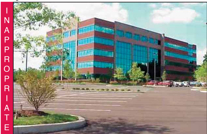
Photo 11.12—Horizontal ribbon windows and reflective vertical glass curtain wall as shown in this photo are discouraged in the UDO.
