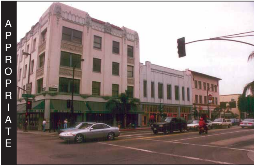
Photo 11.8—The buildings above meet the design standards which require 75 percent of the exterior facade (excluding windows, trim, and doors) to be covered in a durable, attractive masonry material.
