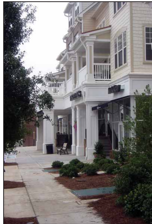
Photo 11.14–The roofed balconies of these second story residential units extend out past the building facade and help to create a sheltered entry to the retail on the lower level.
