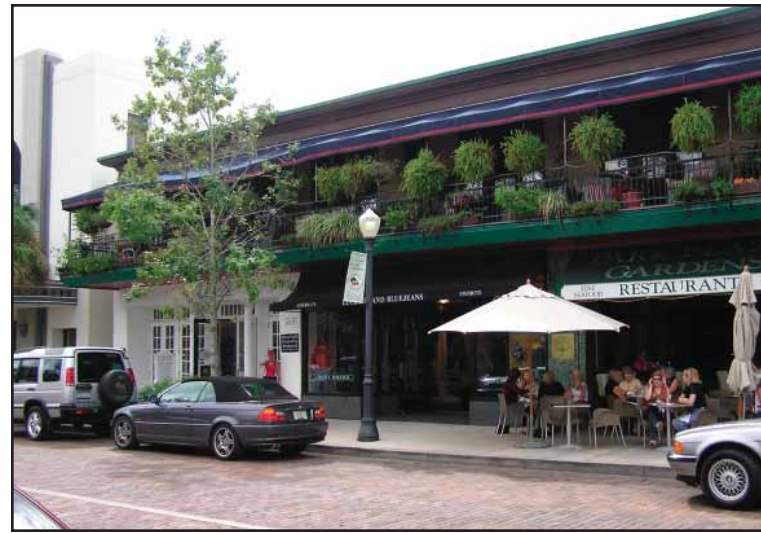
Photo 11.13–A second level restaurant balcony is covered by a large awning. This balcony would be permitted to be enclosed from December through March subject to the approval of the planning staff.
