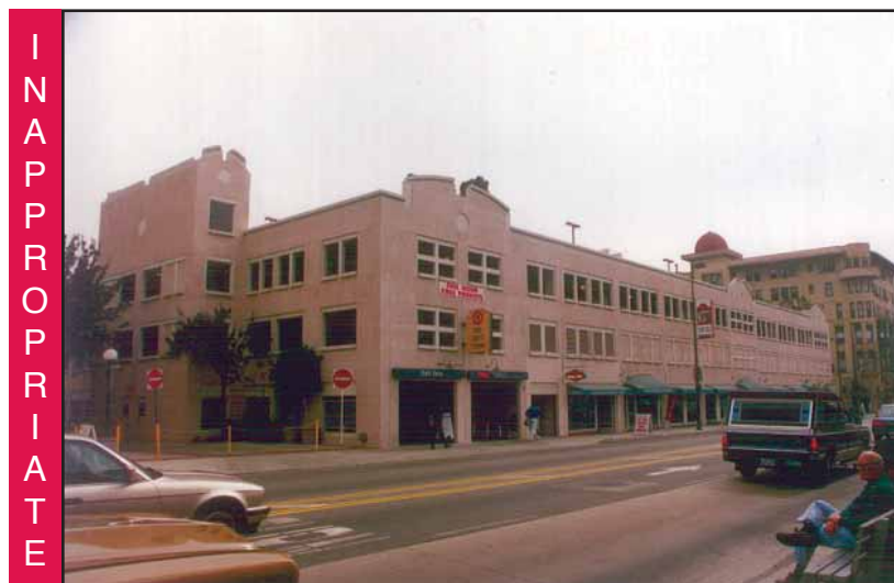
Photo 7.3—While an attempt has been made to provide ground level retail and minimize the “garage” appearance of this parking structure, the overall facade is too repetitive and does not achieve the goals of the development standards.
