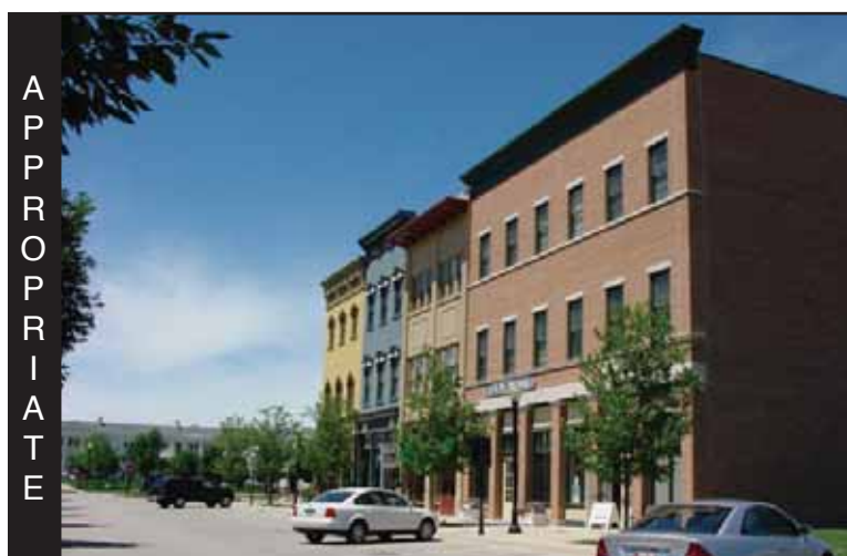
Photo 6.4—Although this building has contiguous frontage along the street edge, it is articulated to create the impression of a series of smaller buildings.
