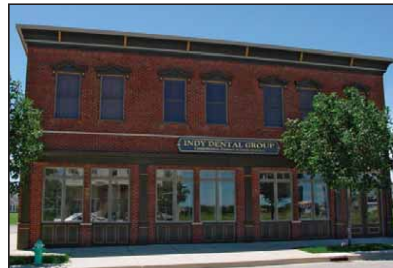
Photo 11.11—The building above illustrates an example of acceptable windows as defined by the guidelines. Individual framed windows cover more than 15% of the wall area and ground floor windows are more than 18" above the finished floor.
