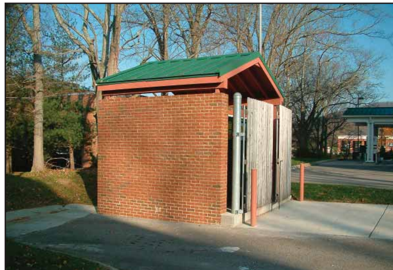
Photo 10.2—Masonry should be the primary material for screen walls at dumpsters and other equipment. When possible, these areas should also be screened overhead to protect views from neighboring uses.
