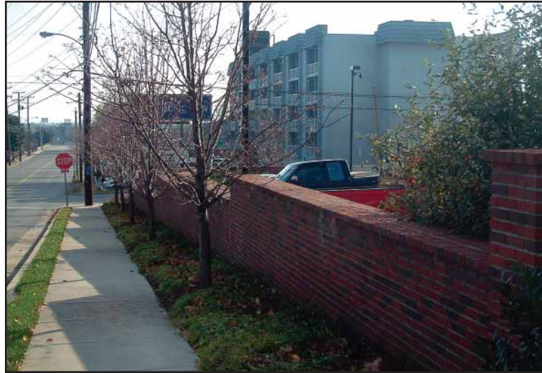
Photo 7.4—Masonry screen walls as shown in the photo above and in Figure 10.1 are required at all sections of surface parking abutting the frontage line of any lot.
