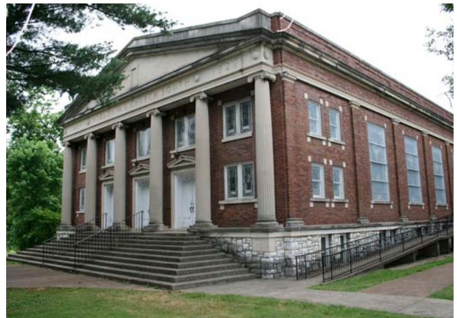
Figure 13: Hobson Methodist Church
