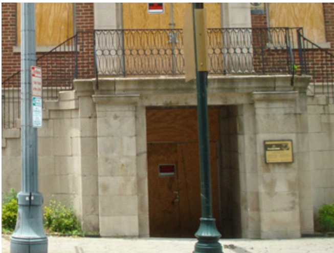
Figure 23. 20-24 Butler Street NE. Abandoned YMCA building. Structure has historical significance as noted at Figure 24.
