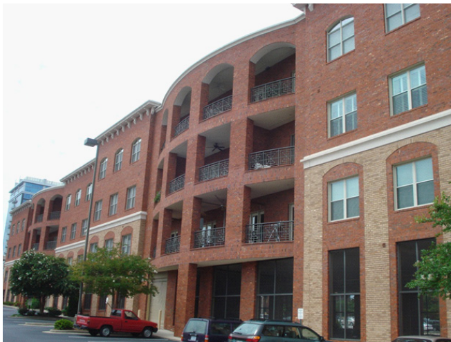
Figure 22. Governors Court Condominiums, 113 N. Church Street, http://www.governorscourtcondos.com/Home_Page.html . Residential property located about one block north of E. Market Street. Structure appears to be less than 10 years old and also appears to be new construction, not a renovation. One of few residential properties in the area.
