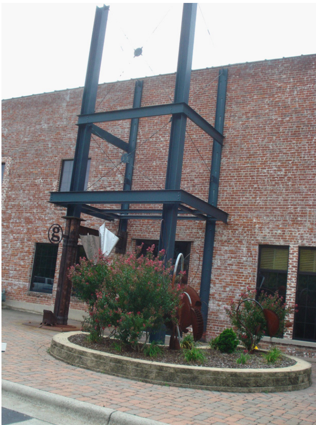
Figure 26A. Refurbished building, 306 E. Market Street. This property rehabilitation is one of many conversions from light industry to commercial.
