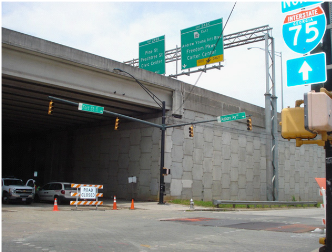
Figure 9. Atlanta Streetcar Project construction near I-75/I-85 underpass at Auburn Avenue @ Fort Street.
