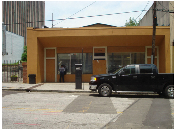
Figure 22. Vacant property on north side of Auburn Avenue NE approximately mid-way between Piedmont Avenue NE and Jesse Hill Jr Drive NE.
