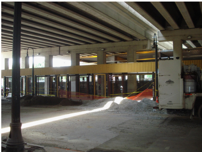
Figure 11. Atlanta Streetcar Project construction on Auburn Avenue at underpass beneath I-75/I-85.
