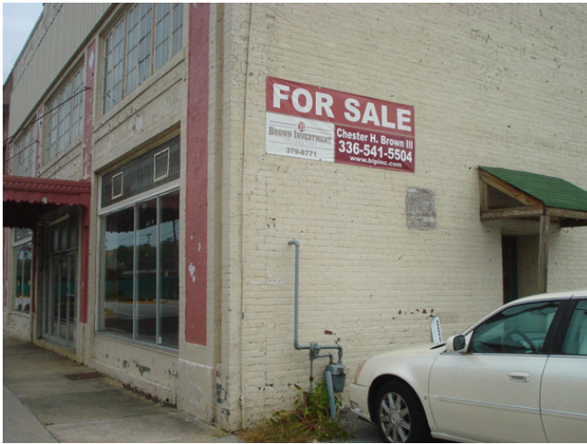
Figure 24. Vacant property, 304 E. Market Street. Property is “for sale,” and will most likely be refurbished for some commercial use, per adjacent properties.
