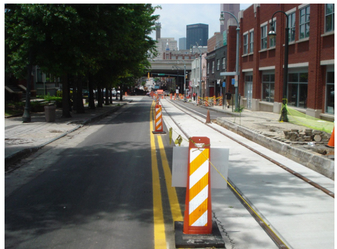
Figure 4. Auburn Avenue looking west. Atlanta Streetcar Project construction has closed off most of the street.
