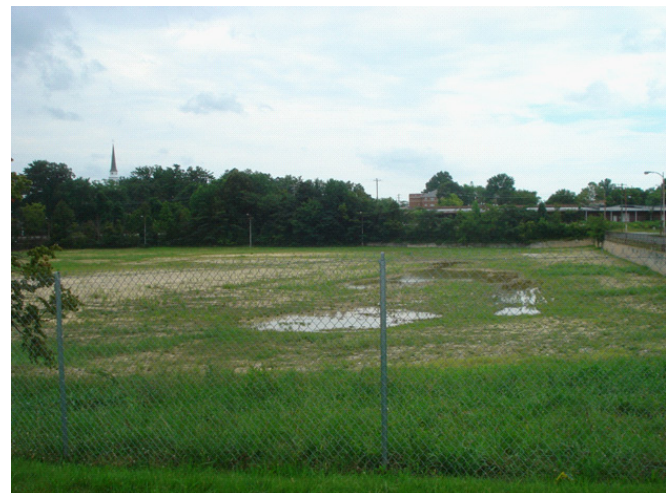
Figure 37. Very large vacant property, E. Market Street (800 block) & Pastor Anderson Street. Property is at least 400-500 yards in length along the southern side of E. Market Street. Uncertain of the land use history of this large lot. It could have environmental issues preventing it from being developed (i.e. brownfields site).
