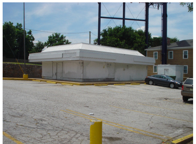
Figure 20. Hilliard Street @ Auburn Avenue – One of many abandoned properties along Auburn Avenue
