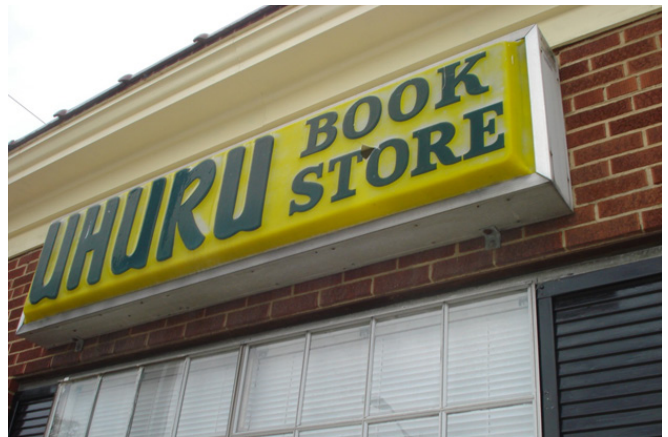
Figure 30. Uhuru Bookstore, immediately west of 418 E. Market Street. Store appears to be closed, permanently. The business next door is closing. Unlike the establishments in the mini-mall, these businesses seem to be doing poorly.
