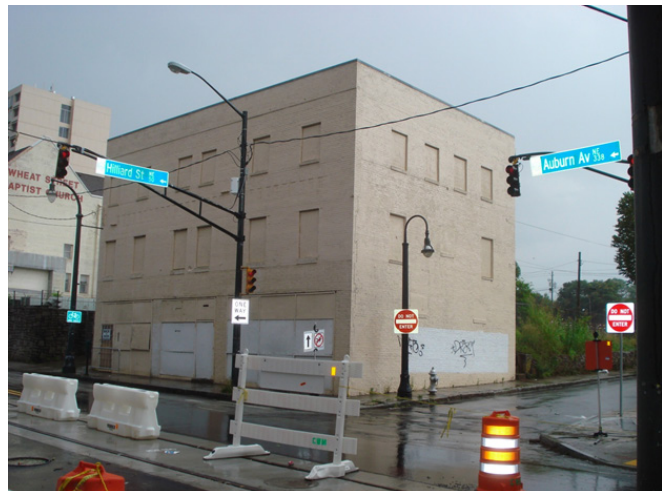
Figure 28. Abandoned building. Hilliard Street NE @ Auburn Avenue NE.
