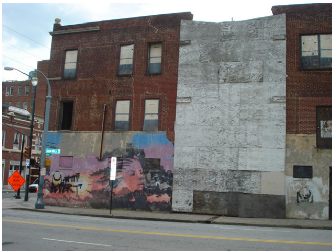
Figure 27. Abandoned buildings. Auburn Avenue NE @ Jessie Hill Jr Drive NE.
