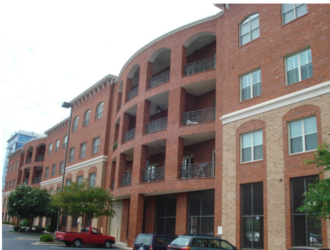
Figure 22. Governors Court Condominiums, 113 N. Church Street, http://www.governorscourtcondos.com/Home_Page.html . Residential property located about one block north of E. Market Street. Structure appears to be less than 10 years old and also appears to be new construction, not a renovation. One of few residential properties in the area.
