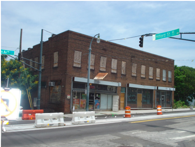
Figure 1. Partially abandoned building – Hilliard Street @ Auburn Avenue (50 Hilliard Street, NE). Construction materials and barriers are associated with the construction of the Atlanta Streetcar Project. Many businesses appear to be struggling to continue to operate during the construction phase.
