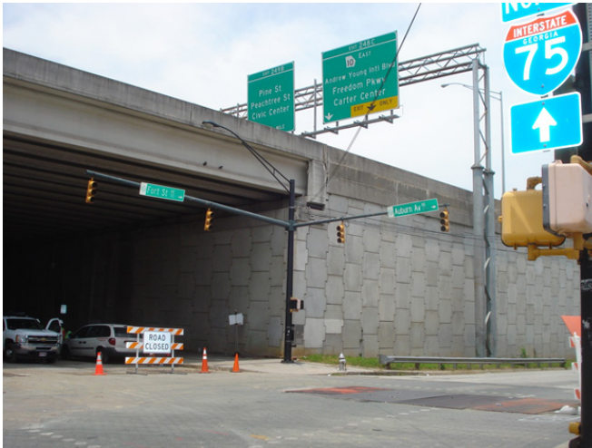
Figure 9. Atlanta Streetcar Project construction near I-75/I-85 underpass at Auburn Avenue @ Fort Street.
