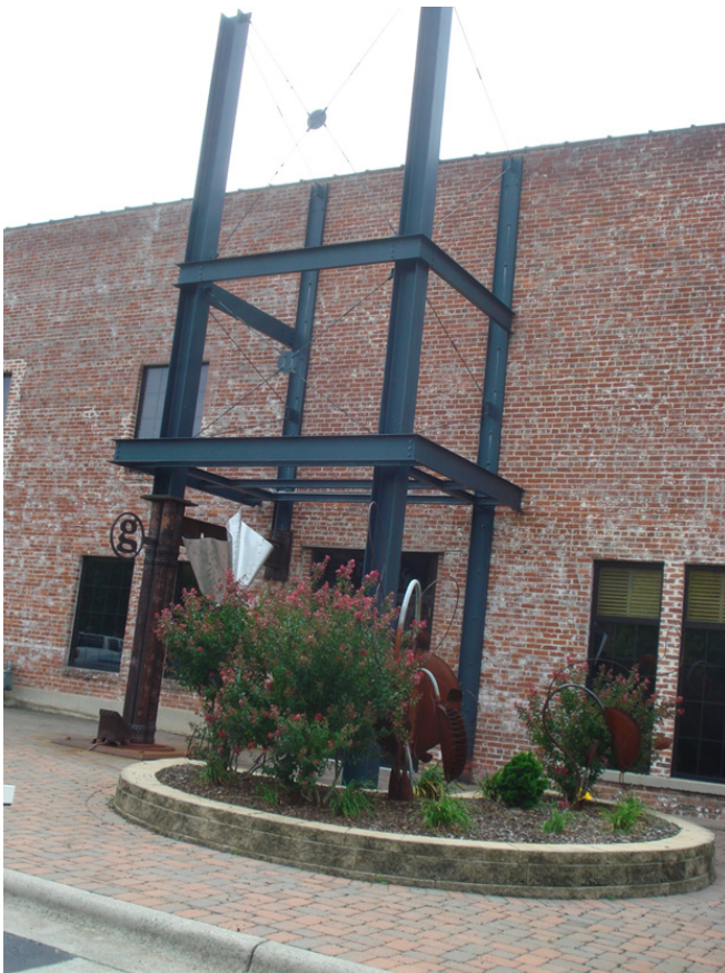
Figure 26A. Refurbished building, 306 E. Market Street. This property rehabilitation is one of many conversions from light industry to commercial.
