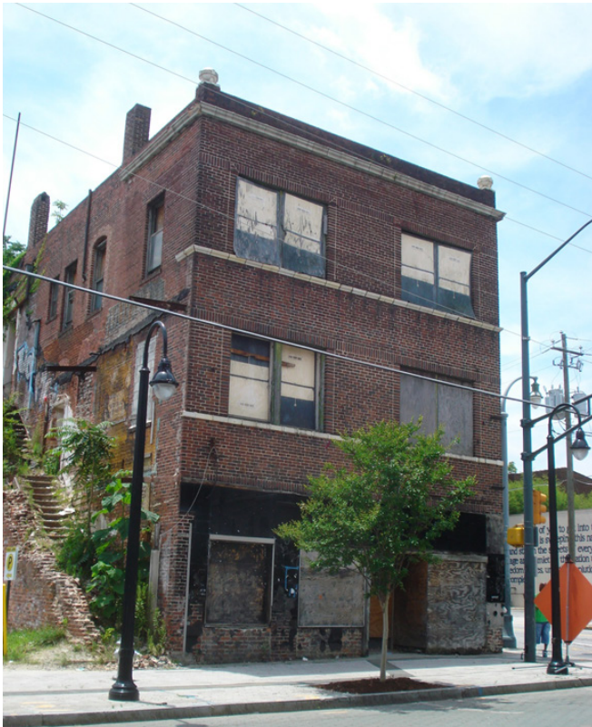
Figure 21. Auburn Avenue NE at Fort Street NE. Abandoned building.
