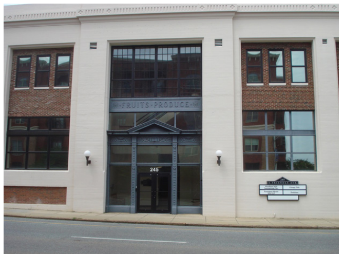
Figure 23. Renovated office building, 245 E. Friendly Avenue, approximately one block north of E. Market Street. Structure appears to have once been a food market per the wording on the façade. One of several examples of refurbished former light commercial and/or industrial property.
