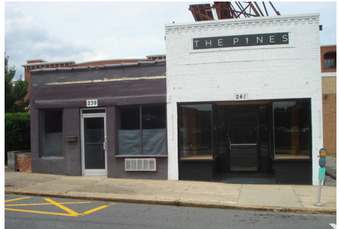
Figure 21. Vacant property, 239-241 E. Market Street. There is increased presence of vacant and under-utilized property as one moves east along E. Market Street towards the North Carolina A&T campus. The properties above appear to recently closed storefronts.
