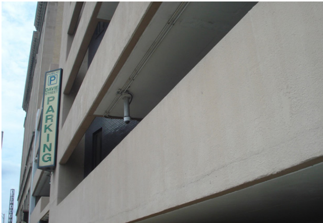
Figure 20. Davie Street Public Parking, E. Market Street & N. Davie Street. One of several large parking structures in the area. The presence of ample off-street parking could potentially support significant future commercial development, and encourage vehicle traffic.
