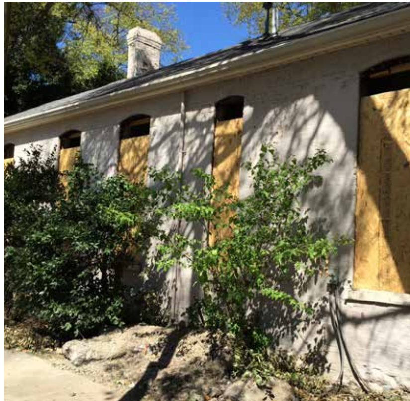
Structure prepped for demolition on Music Row
