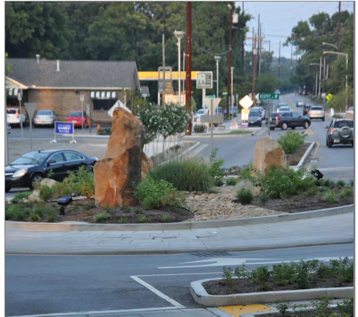
Roundabout located at 51st Avenue South and Murphy Road in Sylvan Park
