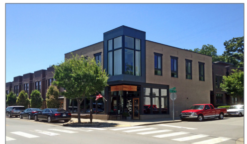
Mixed use building on 12th Avenue South
