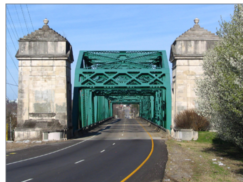
Old Hickory Bridge
