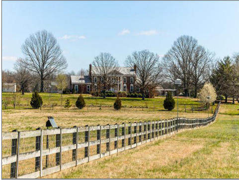
Rural house in Hermitage
