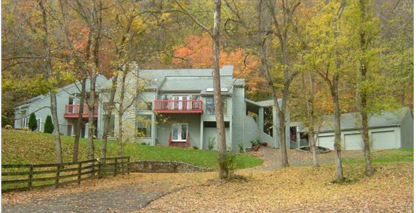
House along Bellevue Manor Drive
