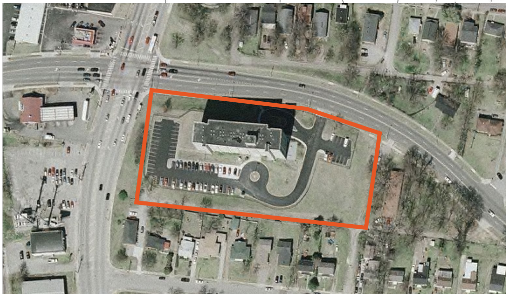
Southeast corner of Wedgewood Avenue and 12th Avenue - existing conditions
