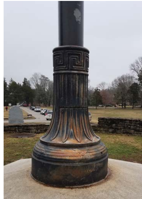
Photo 29 - Flagpole is not in scope, but paint film has weathered, and substrate exposed.
