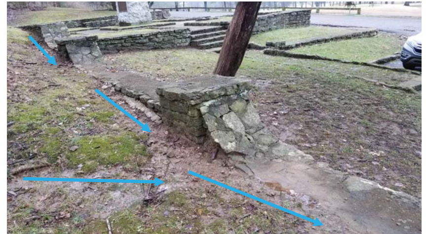
Photo 33 - World War I Memorial path of water from south, moving east, carrying silt
