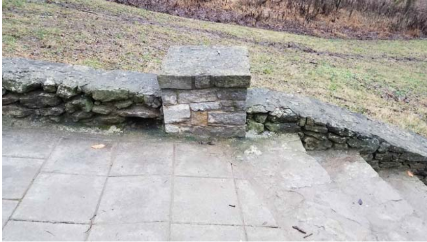
Photo 9 - Pier that was repointed in a previous restoration project in 2001, along with pavers which placed by that project.
