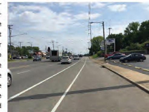
Looking Eastbound on Lebanon Pike East of Central Pike
