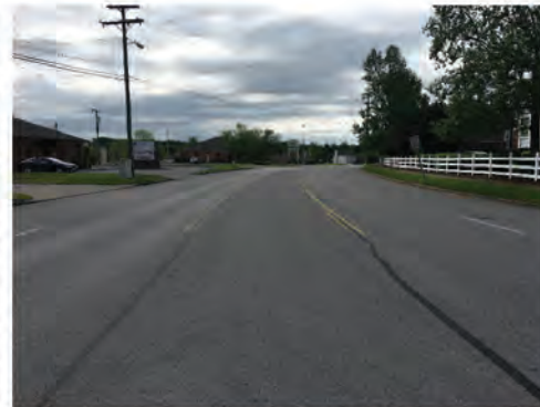
Looking Southbound on Jackson Downs Boulevard South of Lebanon Pike (Western Intersection)
