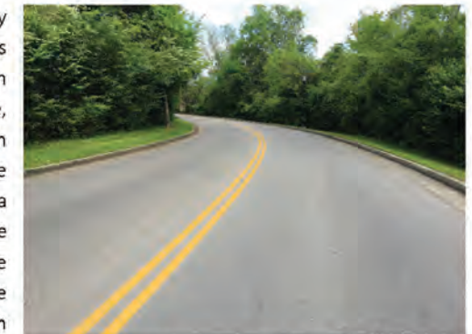
Looking Northbound on Central Pike North of Lebanon Pike
