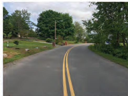
Looking Northbound on Downeymeade Drive North of Lebanon Pike
