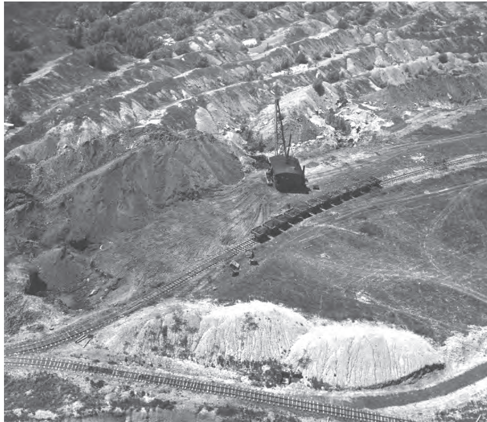
Dragline Phosphate mining near Mt. Pleasant 1939
