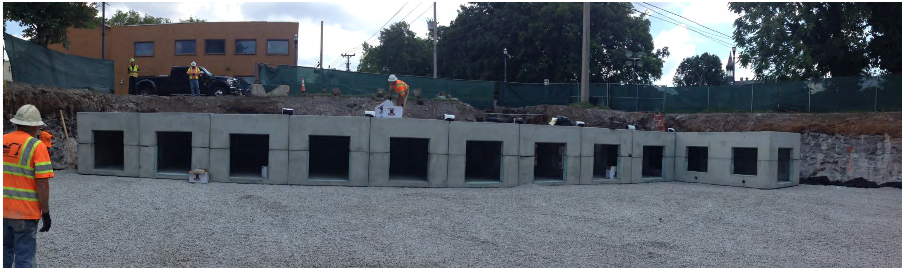
JEFFERSON STREET POCKET PARK UNDERGROUND STORMWATER INFRASTRUCTURE
