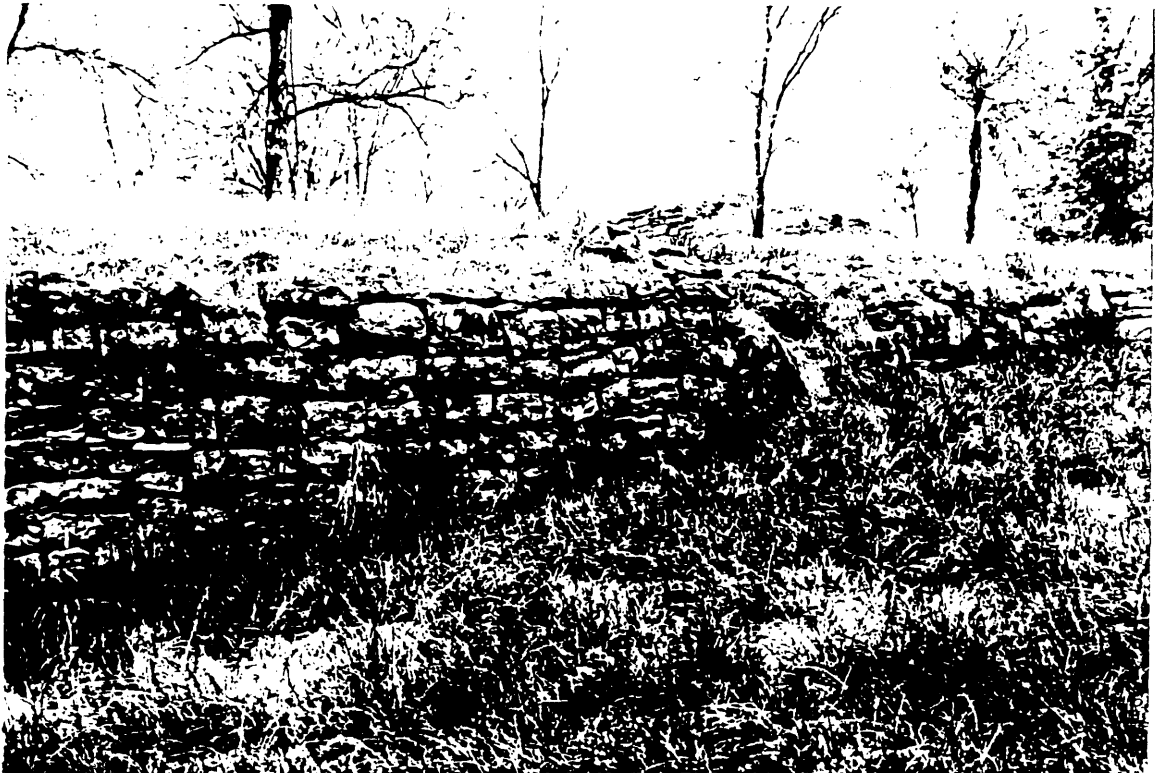
7 Top: Location 17A: bulge and movement. Bottom: Location 18.
