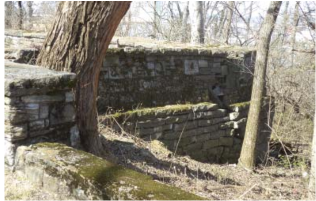
Figure 35. Northeast corner of parking area retaining wall and parapet (JMA, 2013). The loop road wall in the foreground abuts the southeast end of the parking area parapet.
