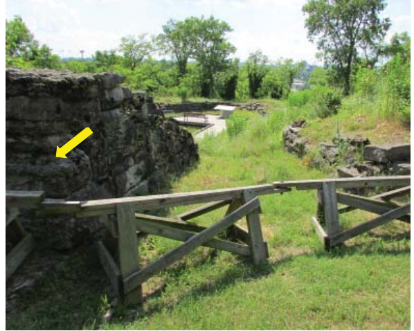
Figure 85 (above left). East Sally Port linking inner works to East Ravelin ditch and East Bastion beyond (1200AE, 2013).
