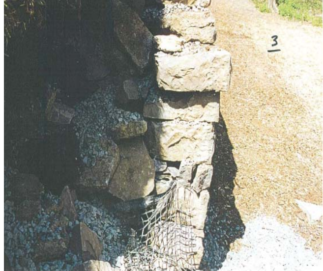
Figure 12. Wall stabilization failure from Geologic Engineering Consultants March 28, 2000, report to Metro Parks and Recreation Board (FNVC).
