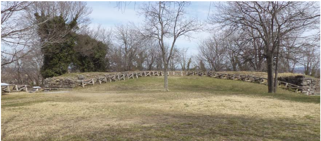
Figure 56 (below). Barricades installed 2004 (JMA, 2013).
