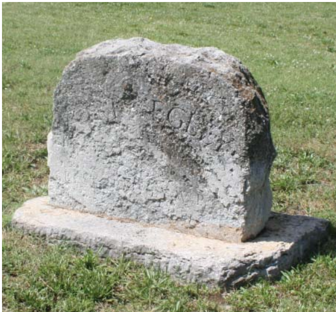
Figure 119. Deterioration of WPA dedication monument (JMA, 2013).
