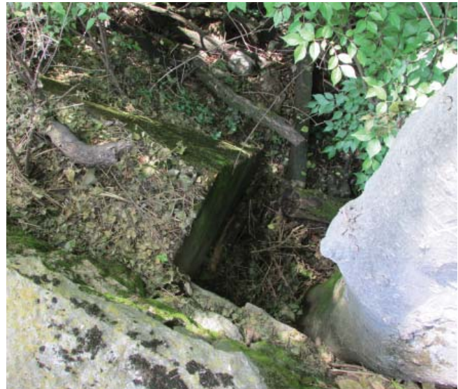
Figure 115. Loss of capstone units and delamination of exterior surface of stones. (1200AE).
