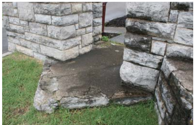
Figure 98. Cracked and broken mortar skim coat on limestone platforms at openings in entrance gate central screen wall, completely missing in some places (JMA, 2013).
