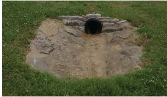
Figure 40. Drainage outlet extending from concrete catch basin inside the loop road (JMA, 2013).
