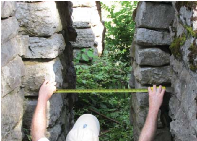
Figure 88. East Bastion tunnel with bulging walls (1200AE, 2013).
