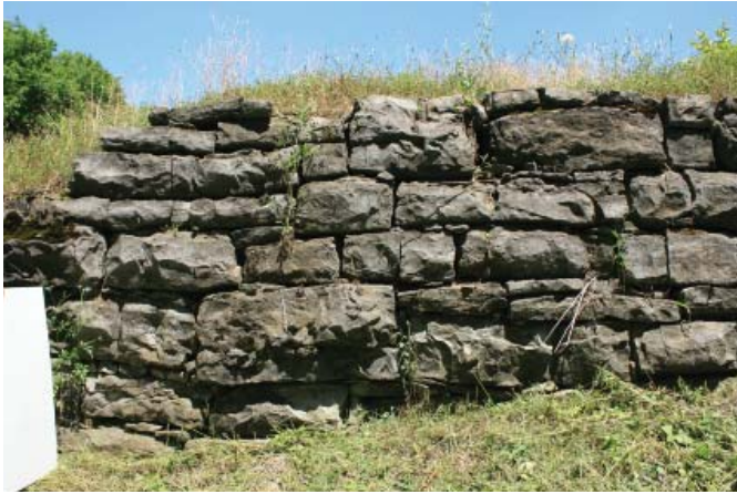
Figure 15. Coursed rough dry-stacked masonry (JMA, 2013).
