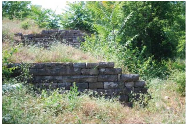
Figure 20 (right). East Bastion, terraced banquettes at southeast corner of the fort (JMA, 2013).
