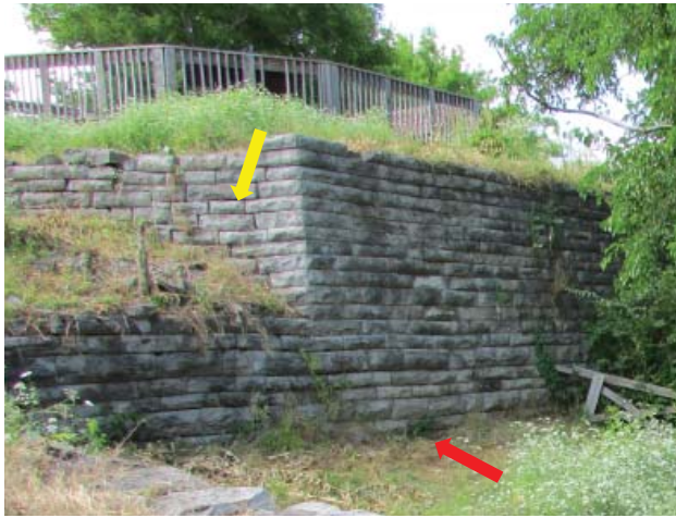
Figure 59. Slight batter—0.03 horizontal to vertical—observed at scarp of South Main Works (1200 AE, 2013).
