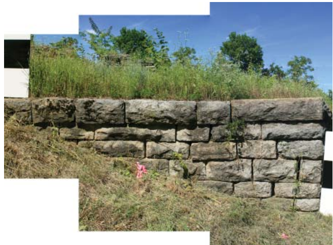
Figure 13. East Bastion, west exterior wall with earth berming (JMA, 2013).
