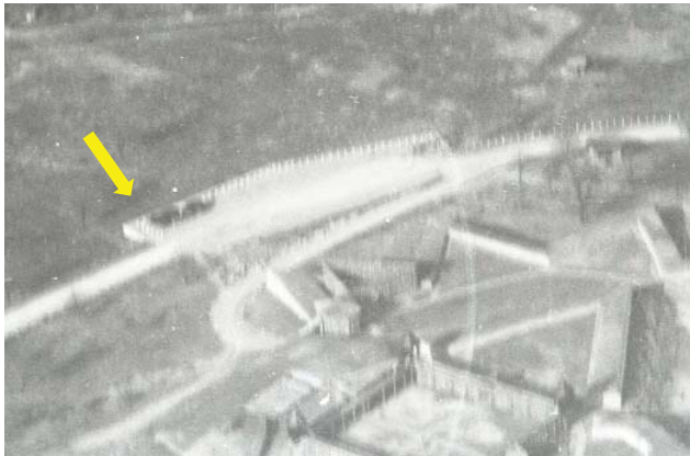
Figure 33a. Fort Negley parking area, November 12, 1936, with bollards or posts edging parking area and outer edge of loop road. Walter Williams, Jr. Collection, Nashville Metro Archives (FNVC).
