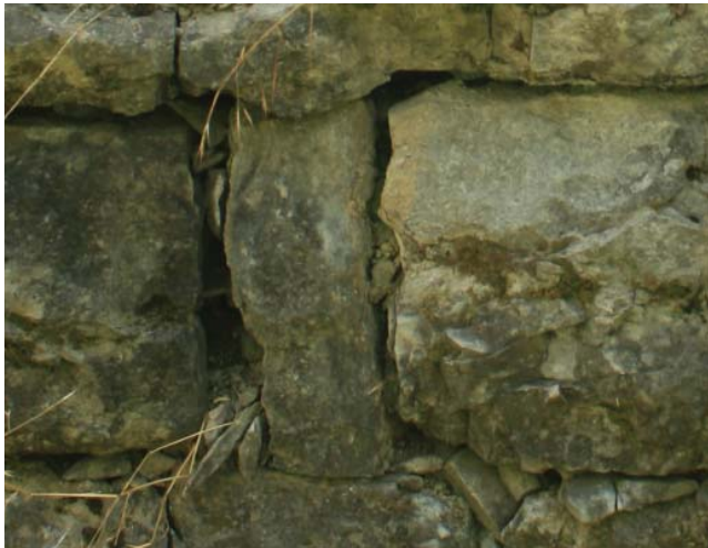
Figure 75. Edge bedded (bedding planes vertical) deadman (JMA, 2013).
