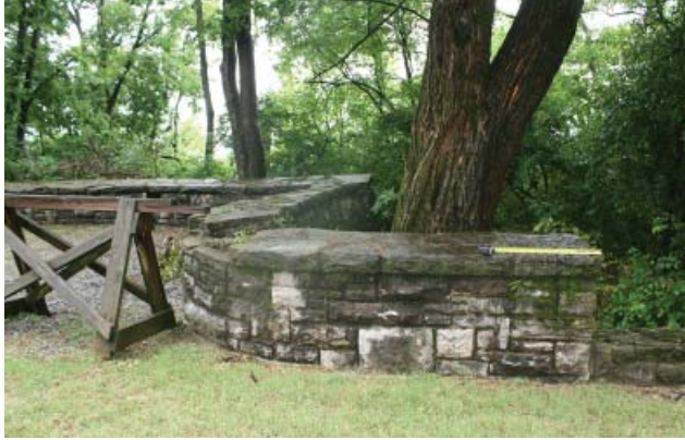
Figure 32. South end of parking area wall (JMA, 2013).
