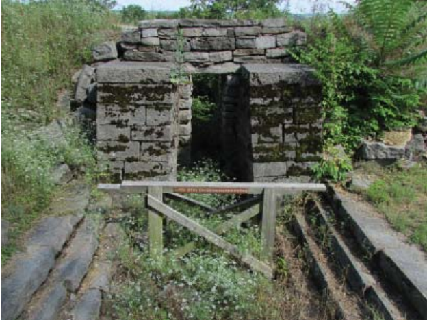
Figure 18 (above). East Bastion Tunnel (JMA, 2013).
