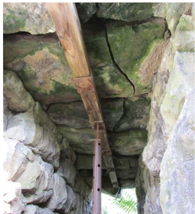
Figure 92. West Bastion tunnel with shoring installed and loss of post shores (1200AE, 2013).
