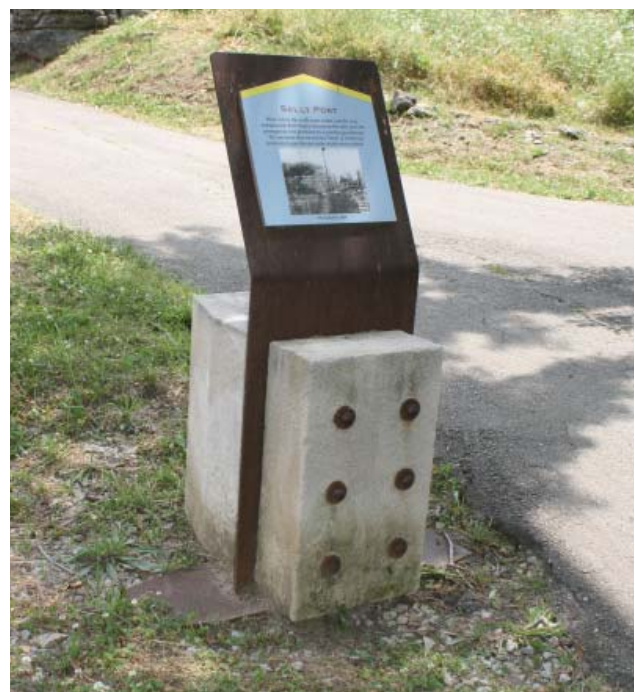
Figure 53. Steel plate with interpretive sign sandwiched between and through-bolted to plinth blocks, installed 2004 (JMA, 2013).
