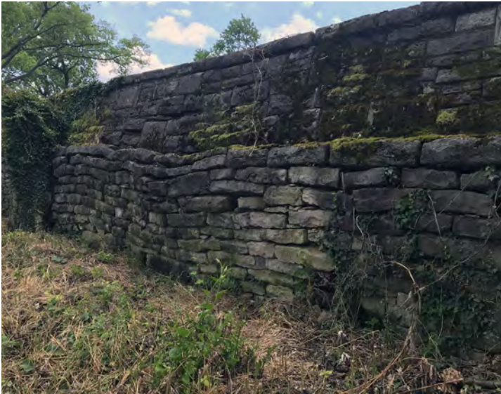
FIGURE 148. A blowout on the northwest corner is due to water runoff and the upper wall's compromising the lower wall. (Encore Interpretive Design)
