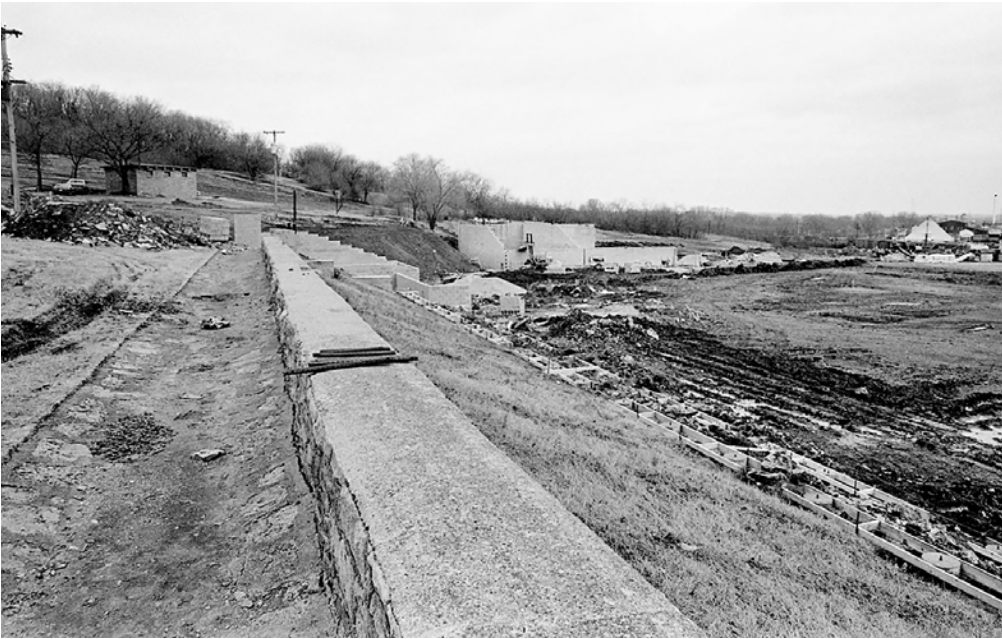
FIGURE 70. The construction of Greer Stadium in December 1977. The footers have been poured for the bleachers and the grandstand is partially completed. Notice the bathroom facility in the upper left corner. It was removed when the stadium was completed in April 1978. (Tennessean, December 23, 1977)
