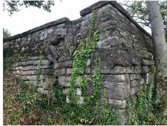
FIGURE 111. Ring road, north parking lot, shows the failing wall due to excessive weight of the cap. (Encore Interpretive Design, 2018)
