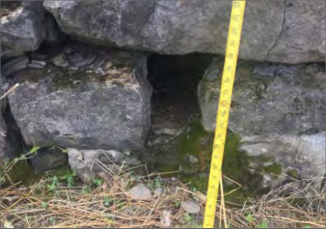
FIGURE 120. Small void at base of exterior wall, Redan Number 2. (Encore Interpretive Design, 2018)
