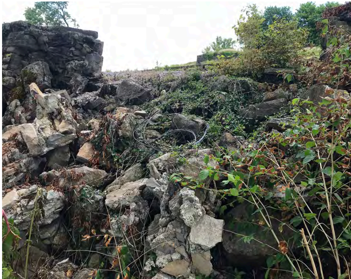
FIGURE 105. The collapsed retaining wall at the ring road parking lot. (Encore Interpretive Design, 2018)
