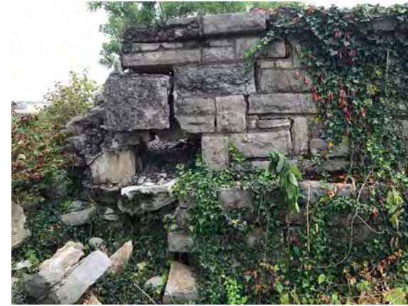
FIGURE 112. Deterioration of cap wall. (Encore Interpretive Design, 2018)
