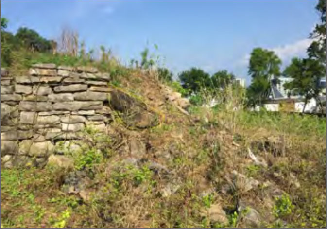
FIGURE 131. Failure of reconstructed wall, Redan Number 7, exterior, south side; note filter fabric marked with yellow outline. (Encore Interpretive Design, 2018)
