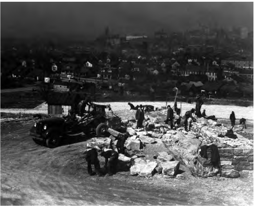
FIGURE 45. WPA workers shaping rock for the reconstruction of the fort in 1936. Union Station, less than two miles away, is in the center of the horizon. (Courtesy of Tennessee State Library and Archives)
