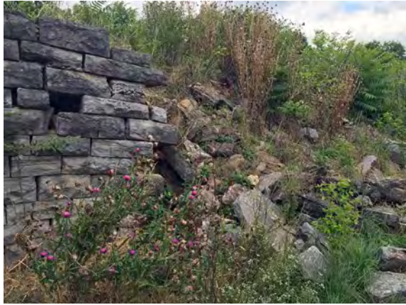
FIGURE 109. Collapsed stonework at the exterior south bastion. (Encore Interpretive Design, 2018)
