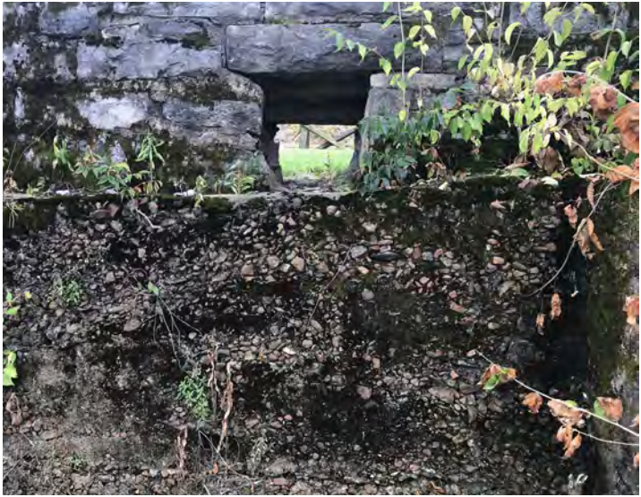
FIGURE 147. The buttressing with concrete has slowed the wall failure. The concrete from the buttress has deteriorated. (Encore Interpretive Design)
