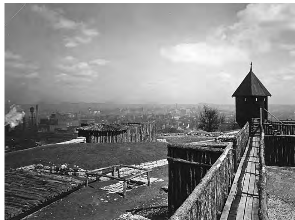
FIGURE 51. WPA Fort Negley Reconstruction c. 1940. The stockade had a platform and turrets for visitors to take in the Nashville skyline. The round roofed structure in the center is the sally port (entrance). In the middle ground with the wooden roof is the museum that visitors entered at the bottom of stone stairs. (Fort Negley Archives)
