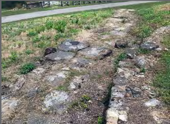
FIGURES 115–116. The stone staircase that leads from the ring road to the sally port consists of large, flat risers. Most of the limestone is cracked, heavily weathered, or missing. (Encore Interpretive Design, 2018)
