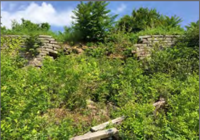
FIGURE 135. New failure since 2013 in reconstructed wall section, south main works, left. (Encore Interpretive Design, 2018)
