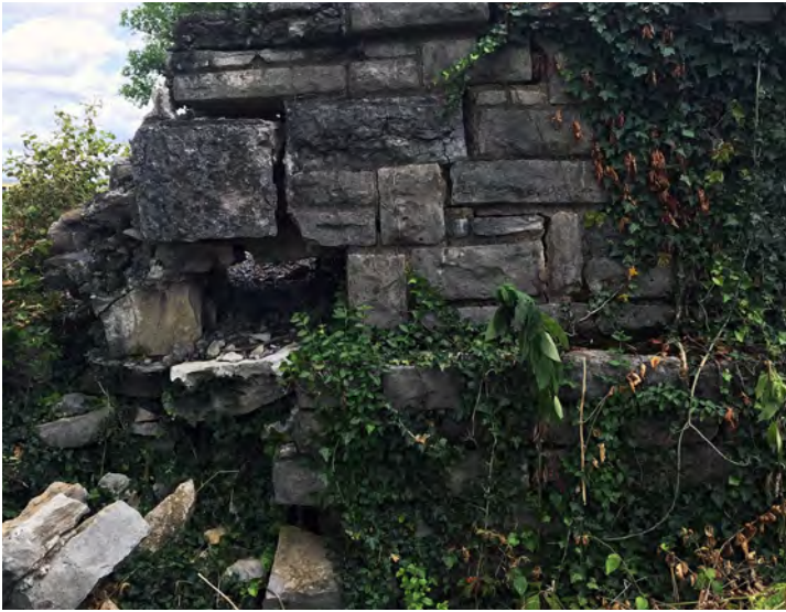
FIGURE 148. A blowout on the northwest corner is due to water runoff and the upper wall's compromising the lower wall. (Encore Interpretive Design)
