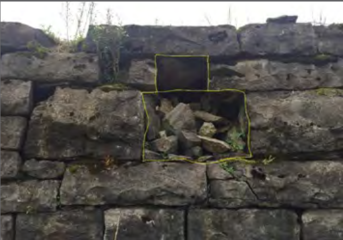
FIGURE 123. Spalls on east exterior side of Redan Number 3 exposing wall packing. (Encore Interpretive Design, 2018)
