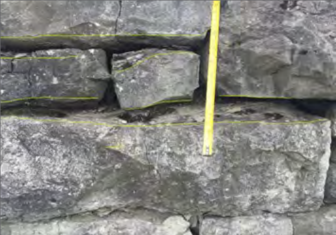
FIGURE 121. Deterioration of shaly limestone at west exterior wall, Redan Number 3. (Encore Interpretive Design, 2018)
