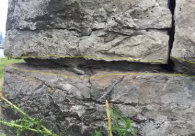
FIGURE 122. Deterioration of shaly limestone at end of west wall, Redan Number 3. (Encore Interpretive Design, 2018)
