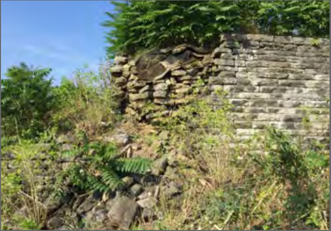
FIGURE 133. Failure of east bastion, east wall, center. (Encore Interpretive Design, 2018)
