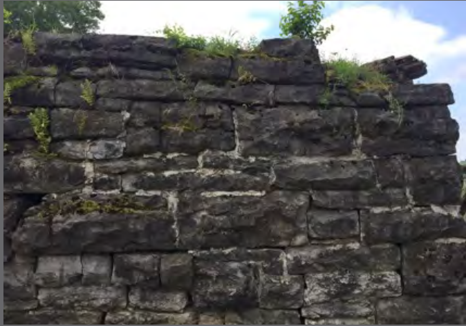
FIGURE 125. East wall facing sally port of the north main works; this wall has experienced bulging and has been repaired by placing mortar in the horizontal and vertical joints. (Encore Interpretive Design, 2018)
