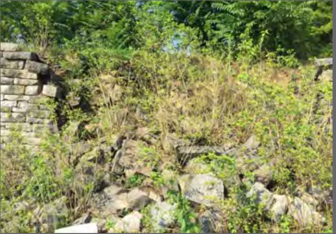
FIGURE 132. Failure of reconstructed east bastion, east wall, right end. (Encore Interpretive Design, 2018)
