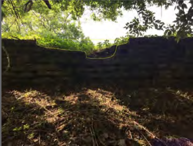
FIGURE 129. Partial collapse, east inner works, exterior, north, right end. (Encore Interpretive Design, 2018)
