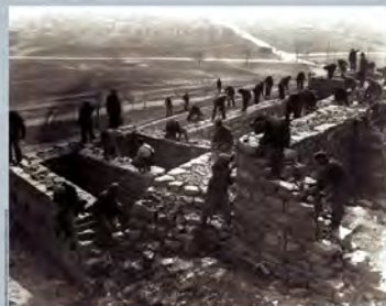
WPA workers reconstructing the limestone walls
