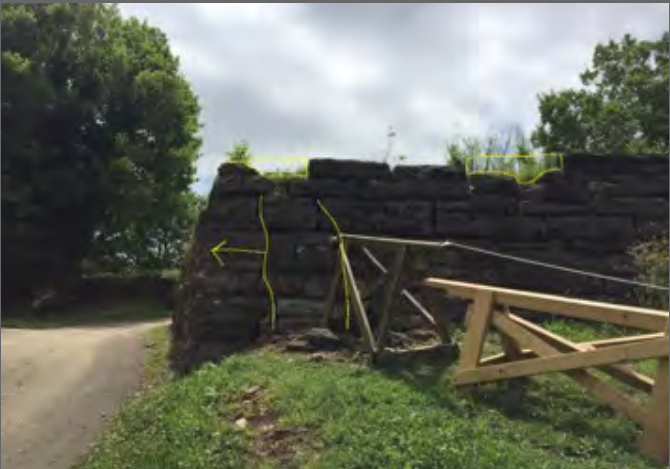
FIGURE 124. North main works, wall has moved toward the left; match with Photo 7; also note missing capstones. (Encore Interpretive Design, 2018)
