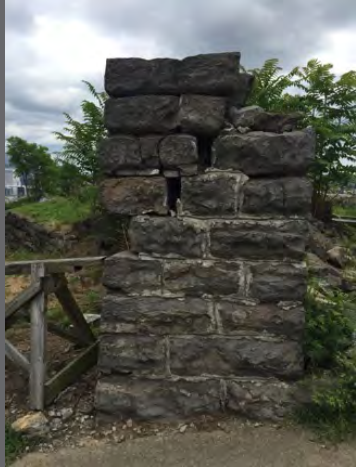
FIGURE 125. East wall facing sally port of the north main works; this wall has experienced bulging and has been repaired by placing mortar in the horizontal and vertical joints. (Encore Interpretive Design, 2018)
