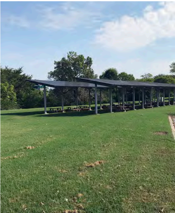
FIGURE 59. The Tennessee Valley Authority operates nine solar arrays around the state. Located north of the parking lot of the Adventure Science Center is a 31-kilowatt facility. (Encore Interpretive Design)
