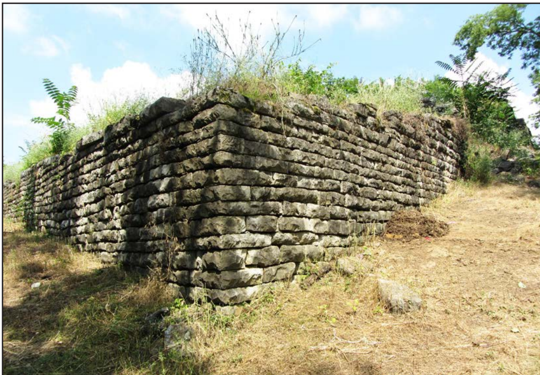
B. Location of Trench 2, Facing Southwest towards the East Bastion.
