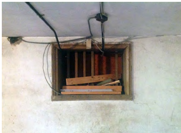
Grilled vents that circulate air in the basement
