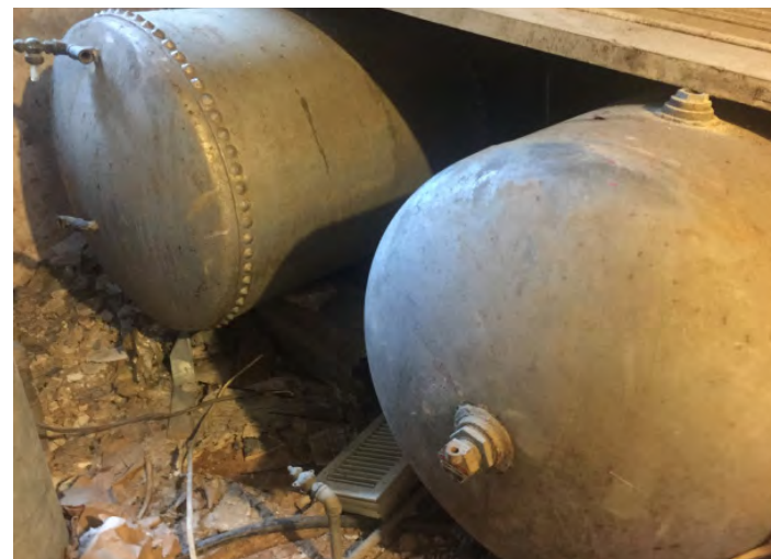
Water tanks in Room 007 once provided steam heat for the radiator system
