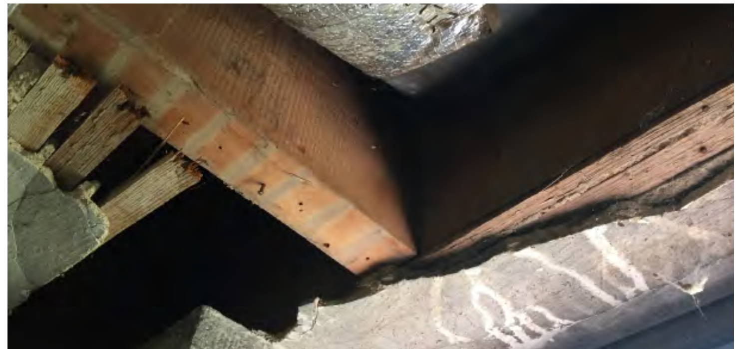
Lathing and plaster issues in the basement of the mansion
