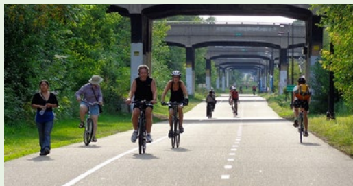
MoZaic in Minneapolis is a mixed use development located adjacent to the Midtown Greenway in Minneapolis. Ramps and stairs connect it to this popular commuting and recreational route.
