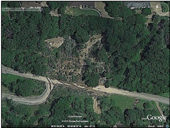
Photo 1: Saxon Drive Landslide
