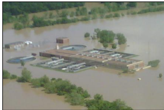
Photo 5: KR Harrington Water Plant
