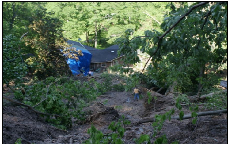
Photo 7: Damage by landslide
