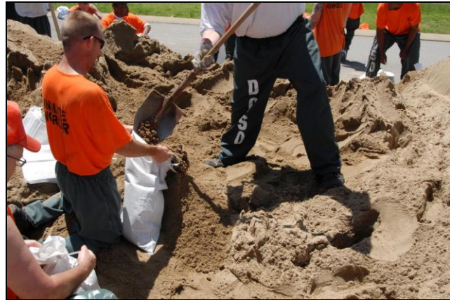
Photo 9: DCSO Inmates sandbagging
