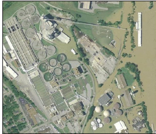
Photo 4: Central Wastewater Treatment Plant
