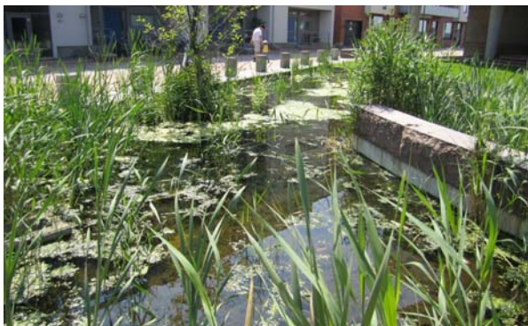
Rain Garden Vastra Hamnen, Sweden
