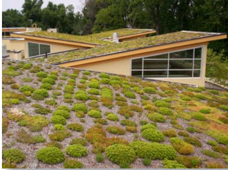
Green Roof at Walter Reed Community Center Arlington, Virginia
