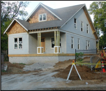
The rise in grade on this lot was not considered, resulting in a foundation significantly higher in the front than what the MHZ approved. Contractors had to stop work in order to devise a solution.
