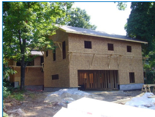
An addition as seen from the alley.
