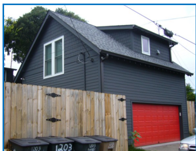
Above: David Baird with Building Ideas, LLC designed the DADU at 1203 Forrest Avenue.
