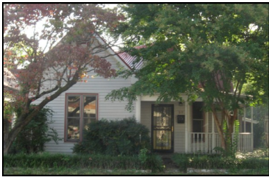
Above: 319 South 11th Street before.
