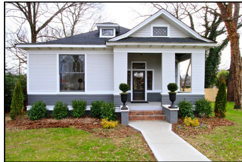
753 Benton received an award in 2012 for its remarkable transformation. The residence required significant repairs for deterioration concealed for decades under faux brick asphalt siding. The original siding was severely damaged and years of neglect and termites had taken their toll on windows and framing.
