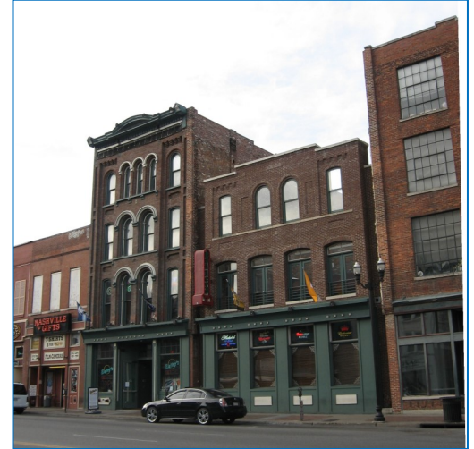
The infill building on this block of Broadway appropriately maintained the established setback and rhythm of spacing.
