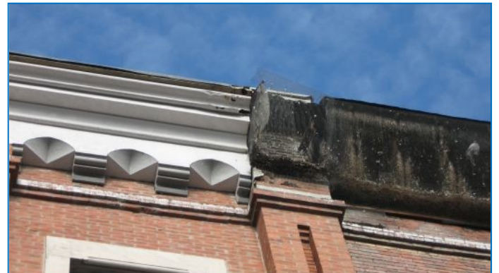
The section of the cornice on the right has deteriorated but originally matched the intact cornice on the left. The missing cornice should be rebuilt to match the existing cornice on the building.
