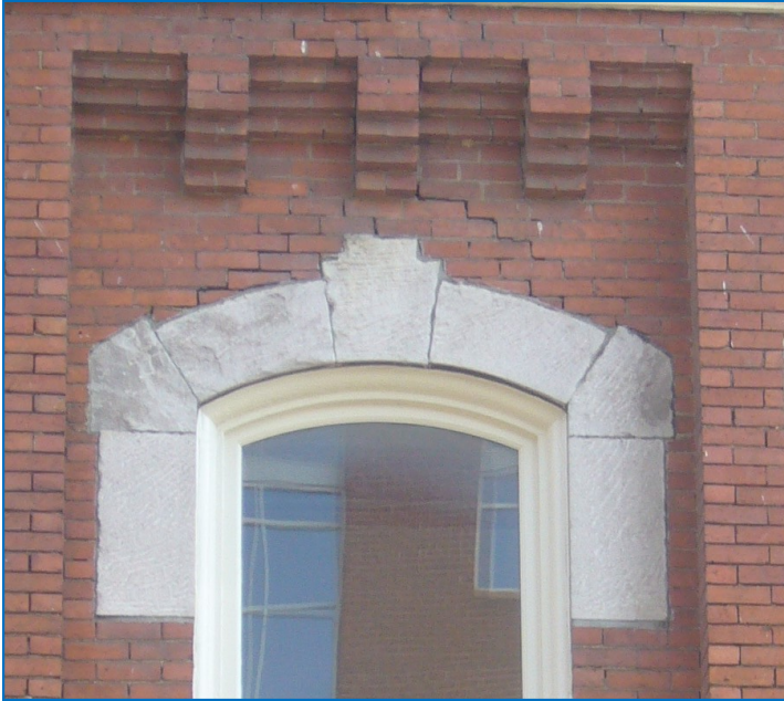
Decorative brick corbelling frames this window.
