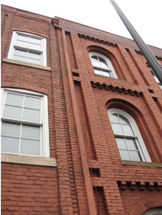
Downspouts on front or side facades should be painted to blend with the paint or masonry color.
