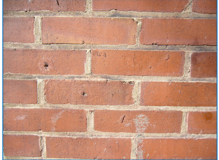
Historic masonry should not be concealed or obscured.
