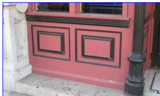
The painted, paneled wood is an appropriate modern bulkhead design.
