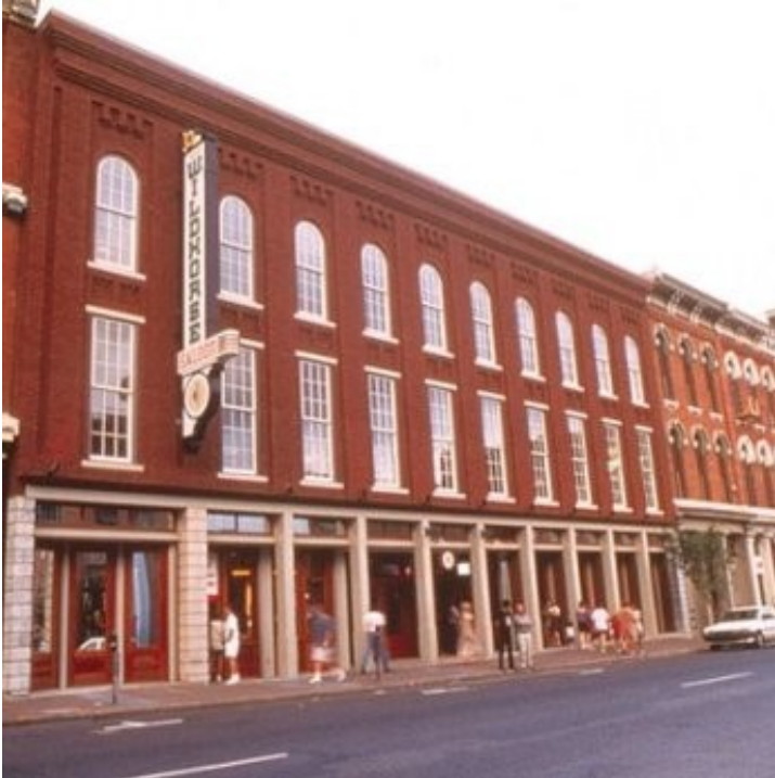
This building was reconstructed based on photographs.
