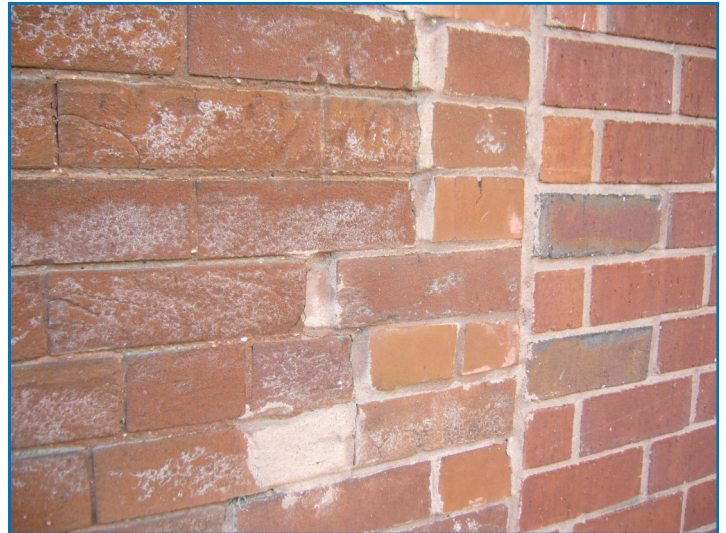
Above is an example of an improper repair that uses bricks of a different color and dimension from the original and the mortar joints also do not match the original tooling.
