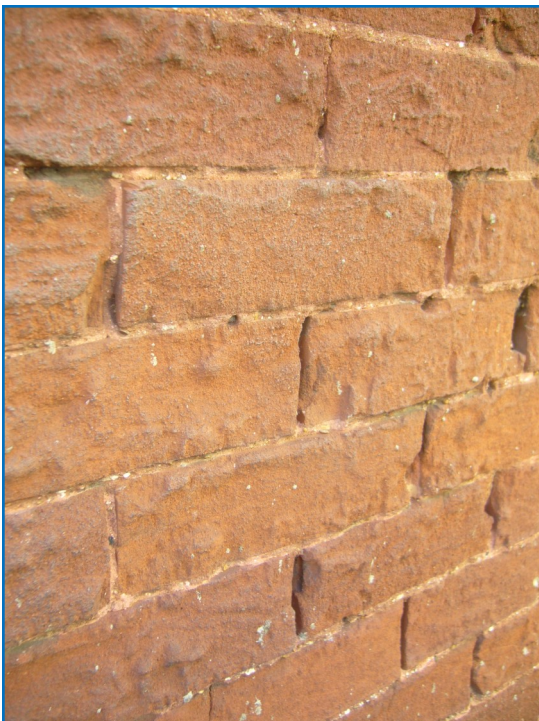
The brick above was cleaned using a harsh method that has removed the hard protective outer surface of the brick.
