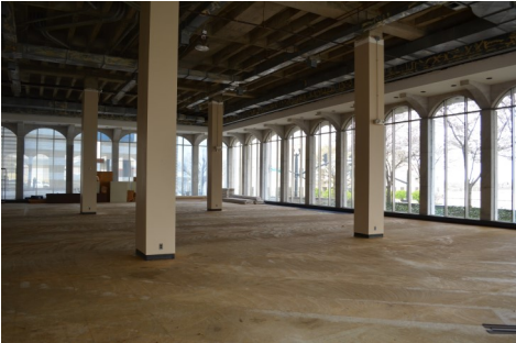
Character defining features of the interior of the Main level of the Ben West Library include the wide open space and arched windows.
