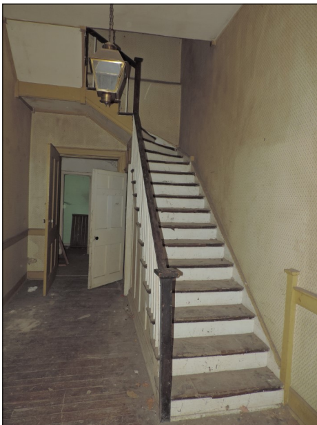
Staircase of the Hall-Harding-McCampbell House at 305 Kent Road, prior to rehabilitation.
