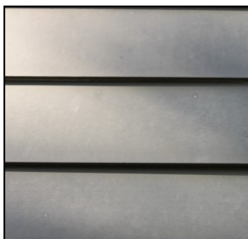
Fiber cement siding is an appropriate cladding for new construction but not when it has a faux (embossed) wood grain, as seen above. Below is an example of a smooth fiber cement siding that looks more like historic wood siding.
