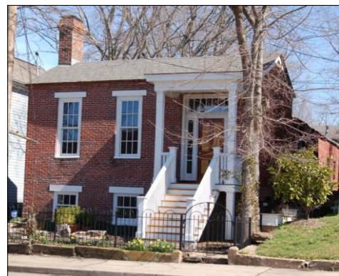
One of Germantown’s oldest residences (c. 1840) on Fifth Avenue North during a renovation.
