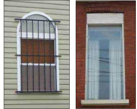
Inappropriate windows alterations.
