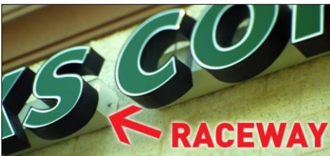
Example of sign with exposed raceway.
