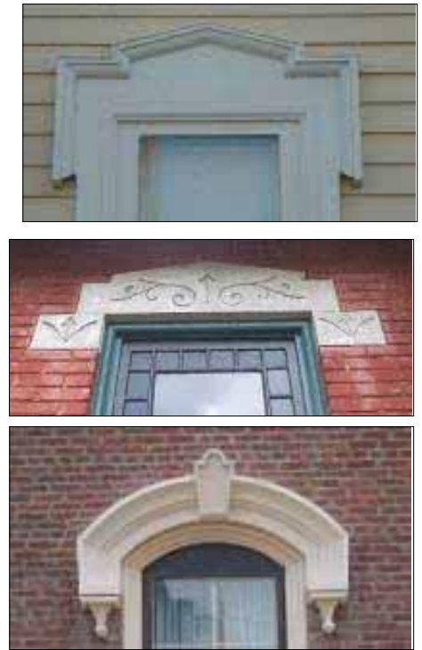
Examples of elaborate window lintels including wood (top), stone (center), and sheet metal (below).
