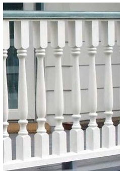
Examples of scroll and saw and turned baluster railing treatments.
