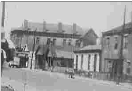
The 1200 block of Fifth Avenue North looking towards Monroe Street (c. 1950).
