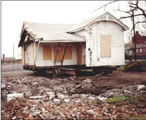
602 Madison Street house prepared to be moved to Hope Gardens.
