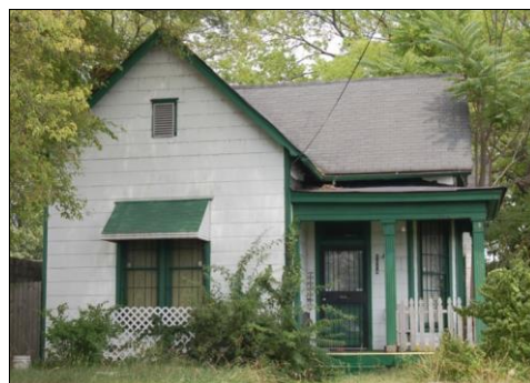
Above: Prior to demolition.
