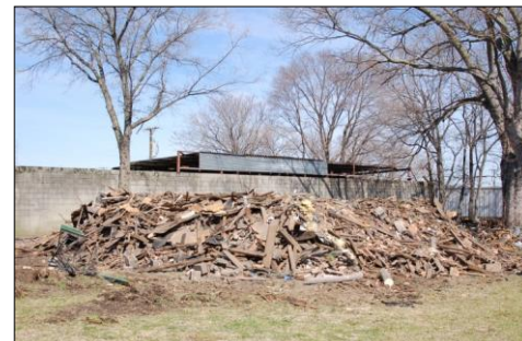
Below: After demolition.
