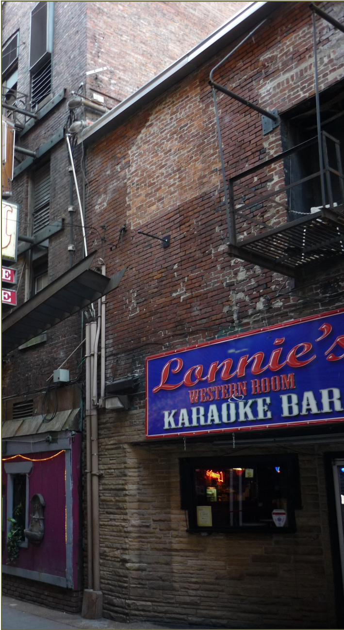
Extremely poor masonry repairs could be a reason for painting brick; although the look could also add to the character of some areas like Printers Alley.
