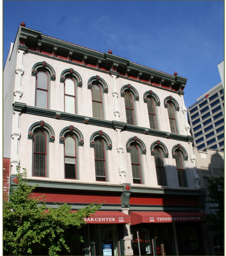
Original one-over-one arched windows at 221 Fourth Avenue North have sheet metal hood moldings. Historic windows and window components should be preserved and retained.
