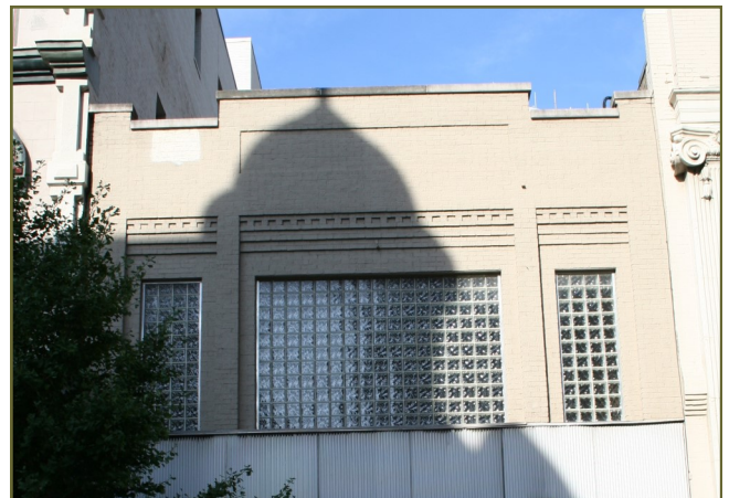
Glass block, such as these windows at 223 Fourth, are a later alteration to the building.
