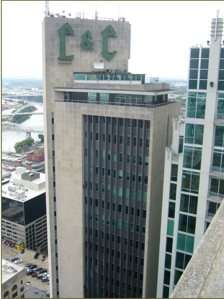
Roofs in the district are primarily flat or appear to be flat with a parapet wall.
