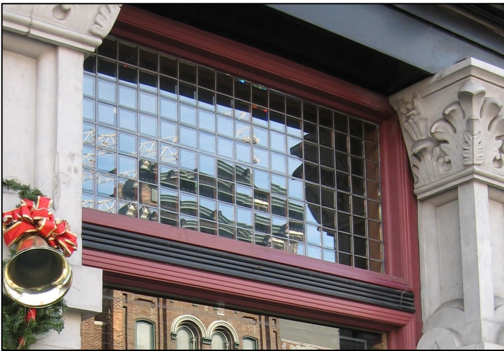
This modern transom on the Merchant's Hotel imitates multi-pane transoms of the turn of the century.
