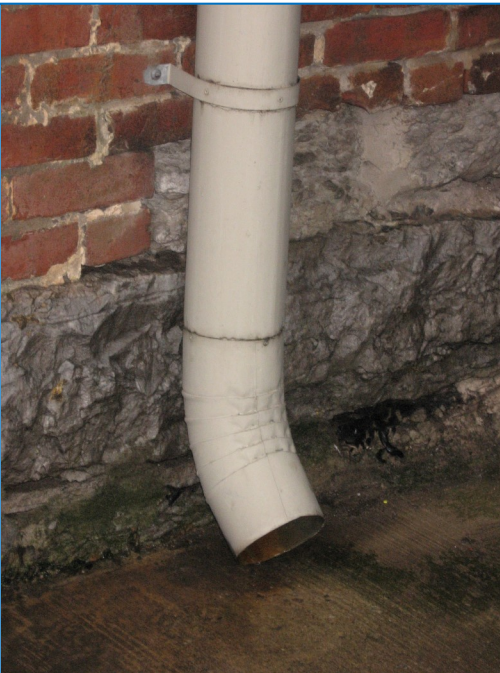
Downspouts should channel water away from the building foundation.
