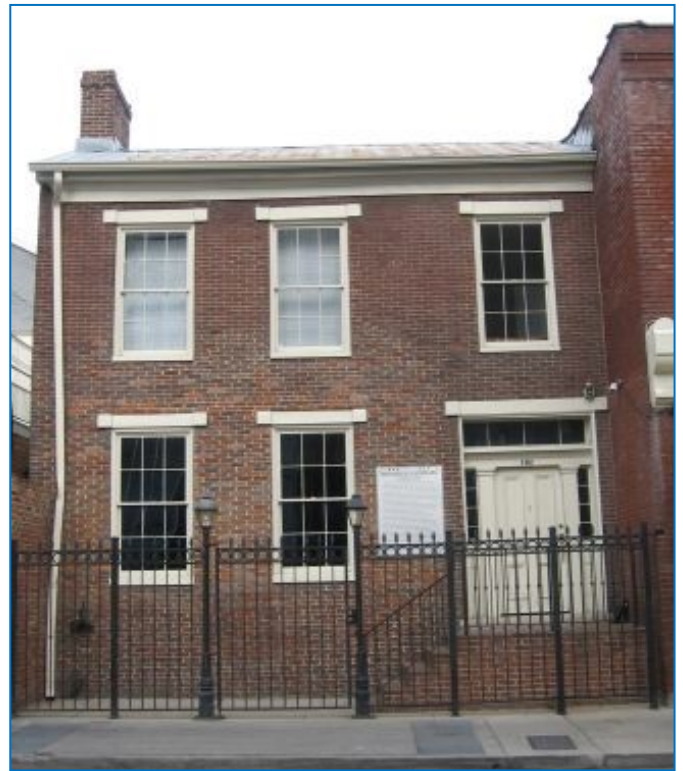
The replacement bricks and brickwork in the lower left portion of this building façade used appropriate bricks, laying pattern, joinery, tooling, and mortaring.
