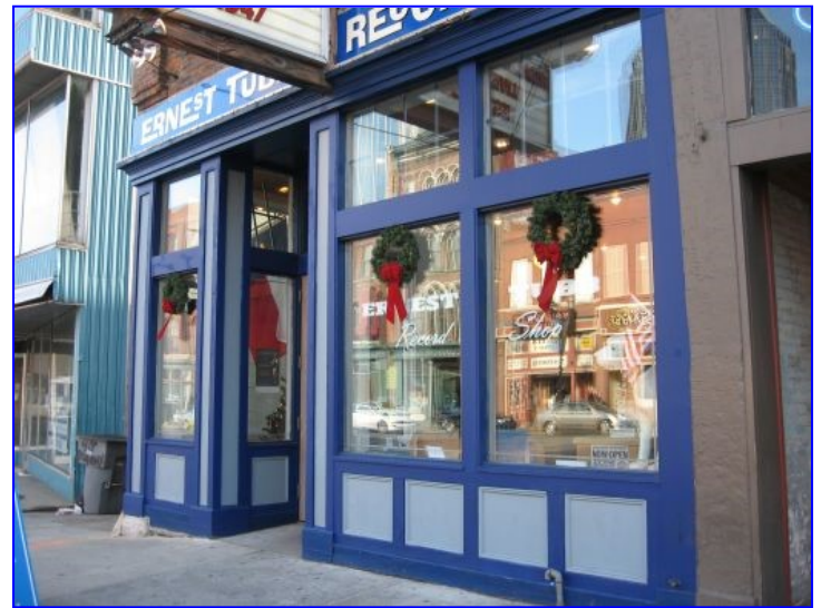
This modern storefront appropriately replicates the missing historic storefront through its incorporation of the typical storefront elements of a recessed entryway, wood-paneled bulkheads, clear glass display windows with wood frames, and clear glass transoms with wood frames.
