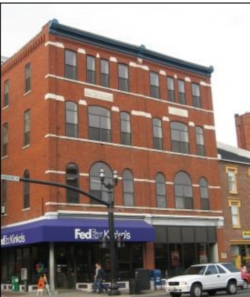
The Broadway Historic District displays a rich variety of upper façade designs from the 19 th and early 20 th centuries.
