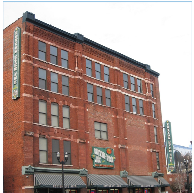
Property owners are encouraged to rebuild missing façade elements such as the bay windows removed on the second and third floors of 200-204 Broadway.
