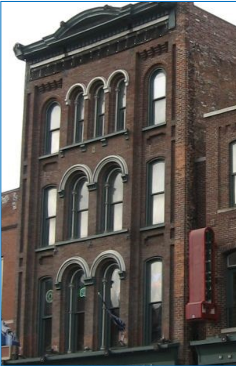
Unpainted stone and brick should remain unpainted unless it was historically painted or if painting becomes needed to preserve the materials.
