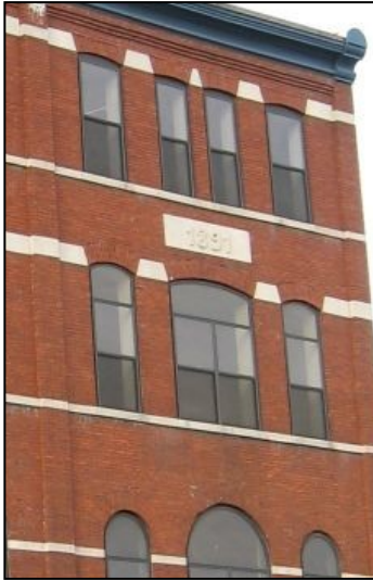
Preserve and maintain historic masonry.
