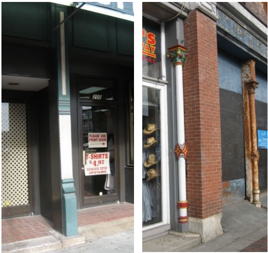
The cast-iron pilasters (left) at 200 Broadway are important structural and design elements to the building. The cast-iron columns (right) are historic and should be retained. The paint used on the left column is appropriate and a good maintenance measure. The column on the right awaits cleaning and painting.
