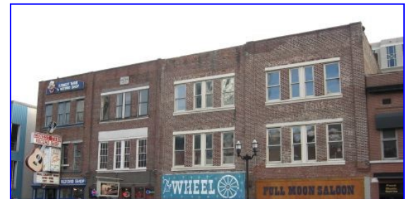
Owners are encouraged to replicate missing cornices where photographic or physical evidence exists. The rebuilding of the historic cornice on this building at 417-423 Broadway as shown below would restore an important design element to the street.
