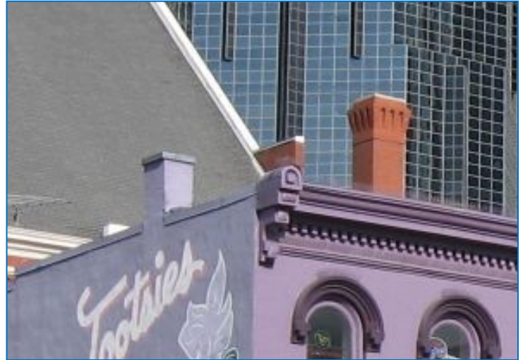
These and other historic chimneys should be retained. They are also appropriate models for replacement chimneys.
