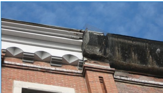
The section of the cornice on the right has deteriorated but originally matched the intact cornice on the left. The missing cornice should be rebuilt to match the existing cornice on the building.
