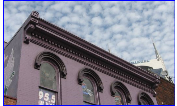
The cornice at 422 Broadway is historic; it should be retained and remain visible. Painting is an appropriate treatment and protects its sheet-metal construction.
