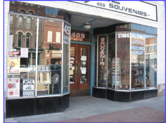
Original display windows like these at 409 Broadway should be retained and, if needed, repaired using materials that preserve their historic appearance.
