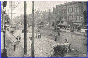
View of lower Broadway c. 1900 showing street paving. The Merchants Hotel is shown in the distance.
