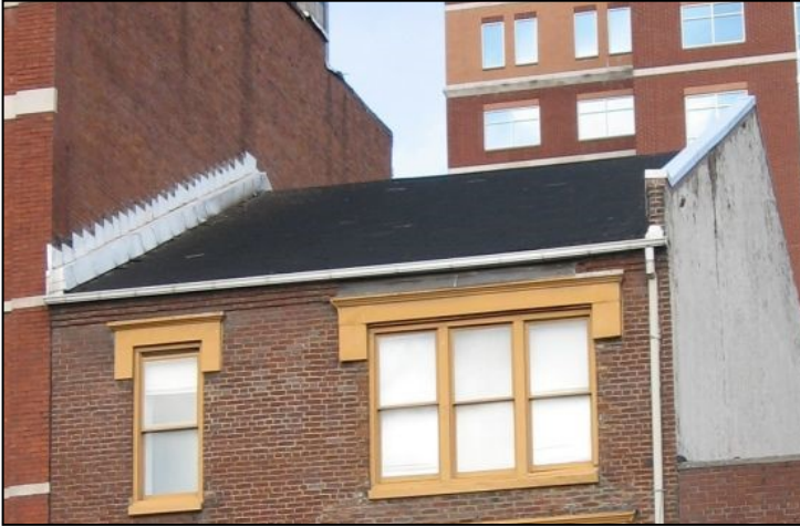
The gabled pitch of this roof is unusual in the district. Its historic pitch and appearance should be retained.
