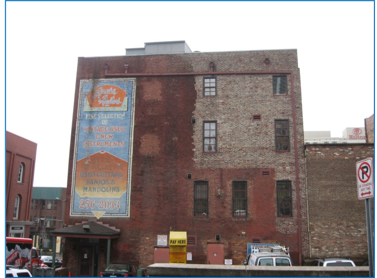
Rear elevations are traditional locations for mechanical units, gutters and downspouts and secondary entrances.
