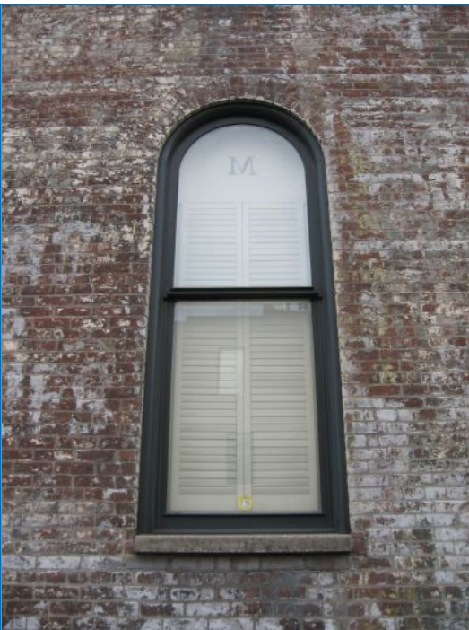
The single-light arched clear-glass panes used in this modern replacement window are appropriate.
