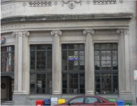
These columns and capitols are historic and an important stylistic element. They and other historic columns and pilasters should be retained.
