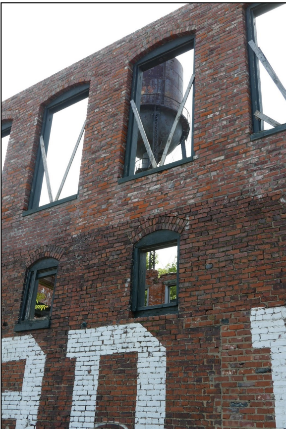
The water tower is a historic feature that adds to the feel and character of the district.
