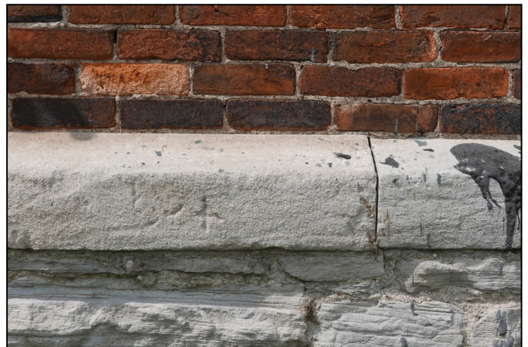
The Mill Building has a stone sill that transitions from the brick wall to the stone foundation.
