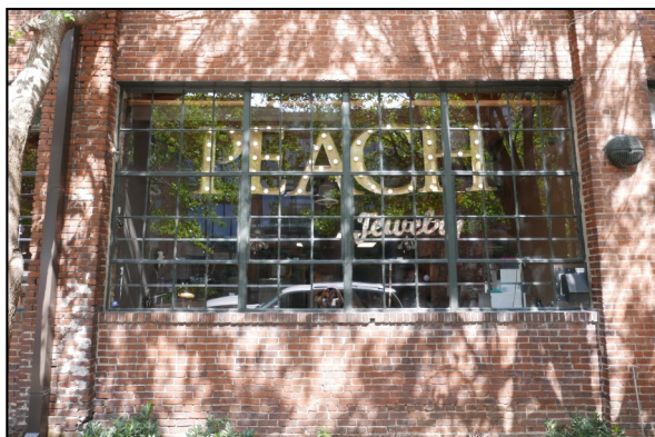
The newer portion of the Mill Building has industrial steel windows..
