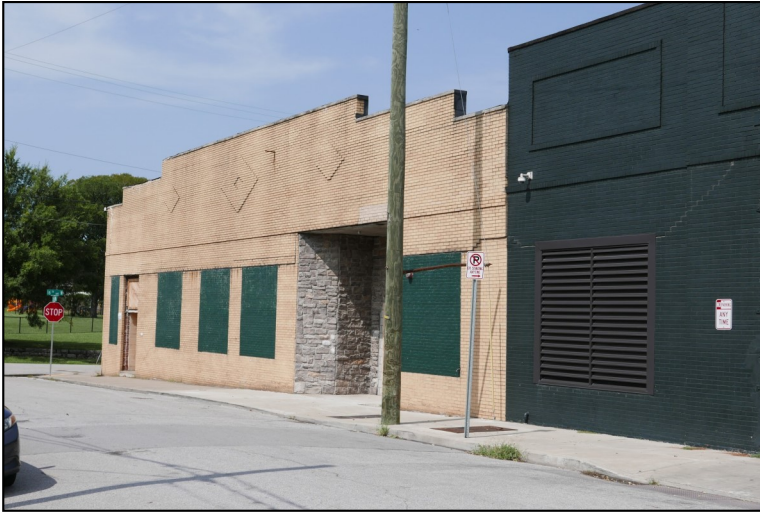
Pitched or barrel vaulted roofs were typically obscured from view with a parapet wall.
