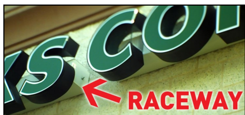
Example of sign with exposed raceway.
