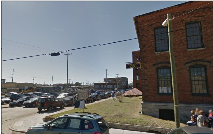
The deepest historic front setback on Clinton Street is 25'.
