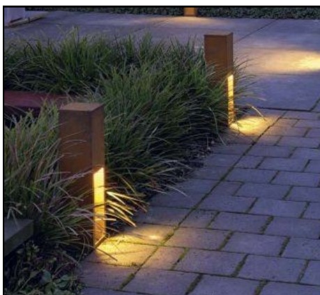
Bollard lighting can be an effective way to provide pathway lighting.
