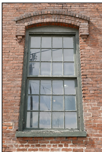
The oldest portion of the Mill Building has wood double-hung windows.
