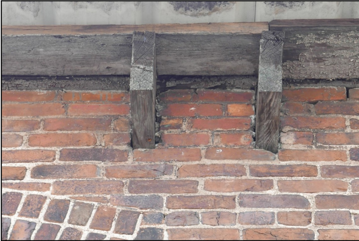
Detail showing the connection between roof and wall at the rear of the Mill Building.
