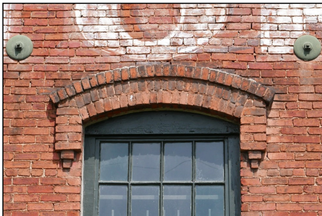
Many historic windows have decorative details that should be retained.
