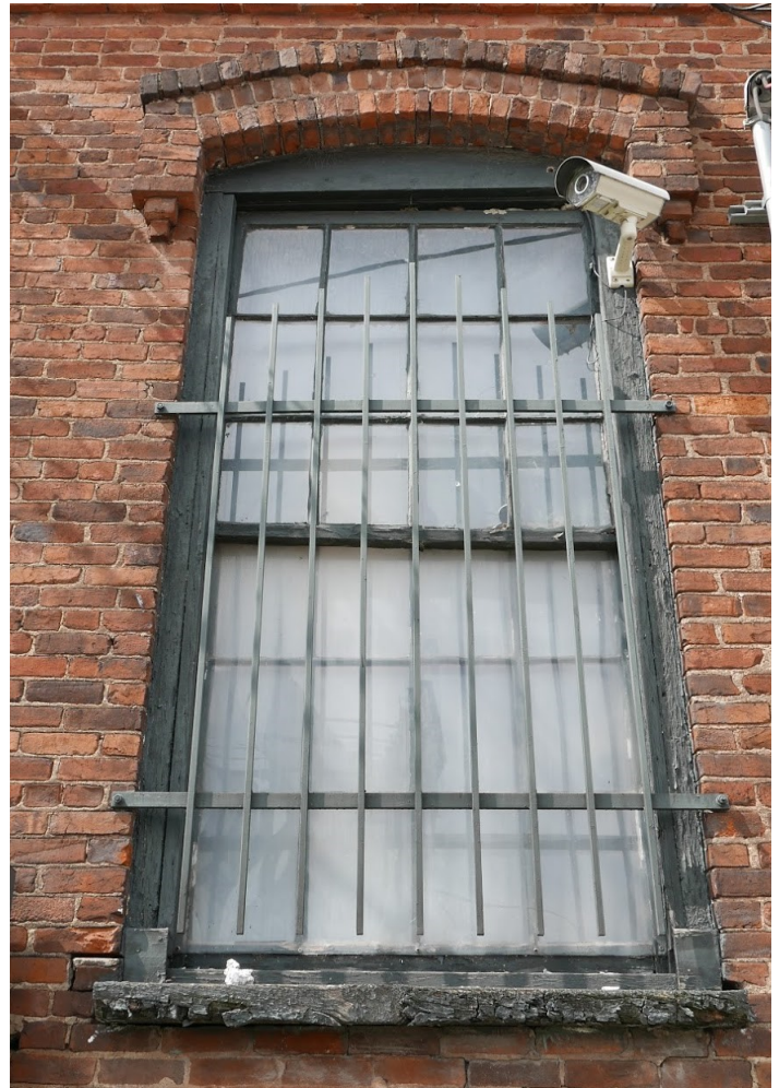
Window bars are appropriate on secondary and rear facades.
