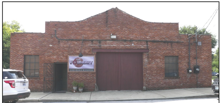
The George M. Fly & Sons building located at 1419 Clinton Street is a contributing building to the Historic Preservation Zoning Overlay.
