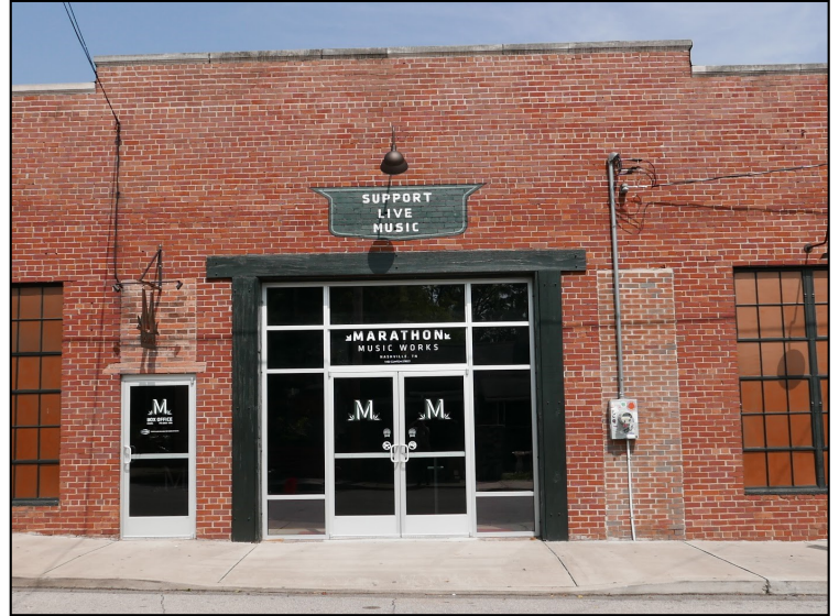
This entrance is an appropriate design for a replacement entrance.
