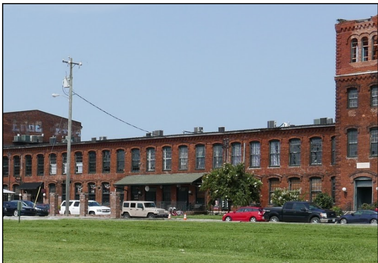
Mechanicals on top of the Mill Building are an example of appropriate mechanical locations as they are not readily visible, except from a distance.
