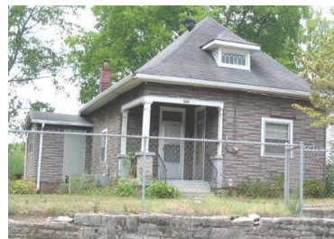
Hipped roof with cutaway porch at 1821 4th Avenue North.
