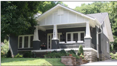
Craftsman bungalows, like 149 Kenner Avenue, is a typical style and form of the district’s early development.
