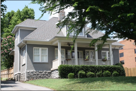
A Colonial Revival bungalow located at 111 Kenner Avenue, with a centrally-located porch, a symmetrical façade, and a roofline is representative of the bungalow form.
