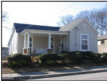
Gabled-ell at 1805 4th Avenue North.
