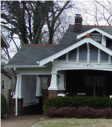
A porte-cochere is a covered entrance wide enough for a vehicle to pass through, typically opening into a courtyard. They are usually attached to the side of a building, one-story in height, and no more than 10'-12' wide.
